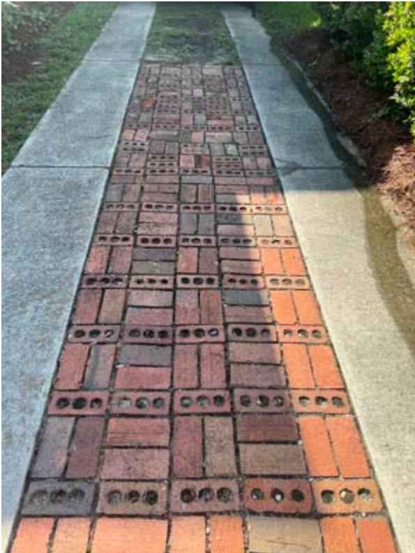
Existing Driveway Brick In-fill
