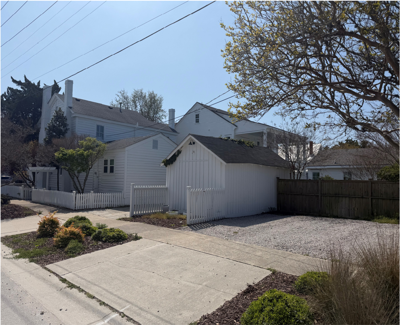
EXISTING VIEW FROM BROAD STREET
