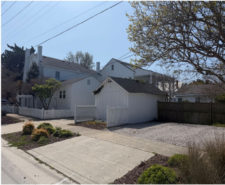
EXISTING VIEW FROM BROAD STREET
