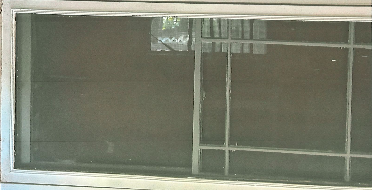
existing window s
