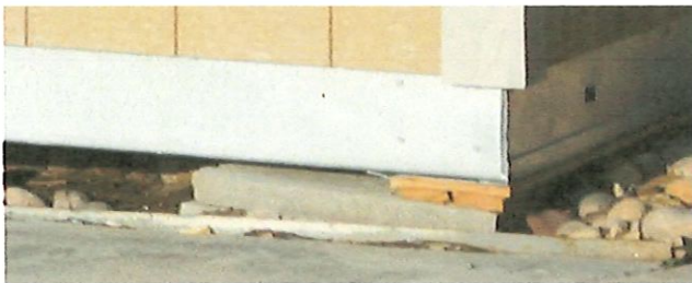
Figure 2 - Close-up of leveling with blocks & shims
