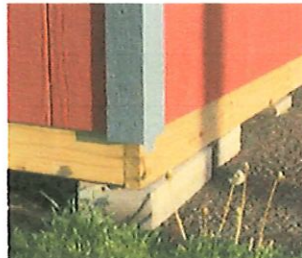
Figure 2 - Close-up of leveling with blocks & shims
