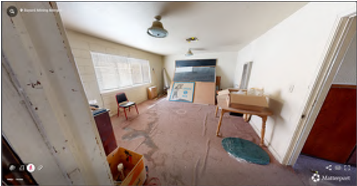
Interior Back Rooms
