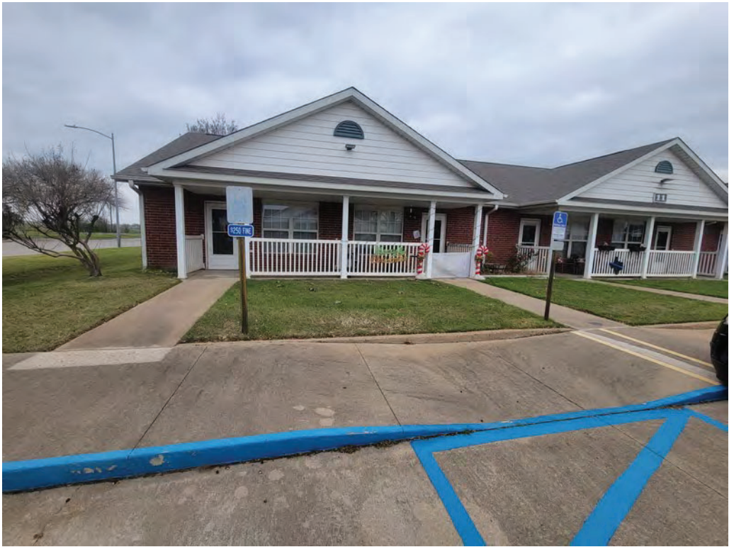
2. ADA parking signage
