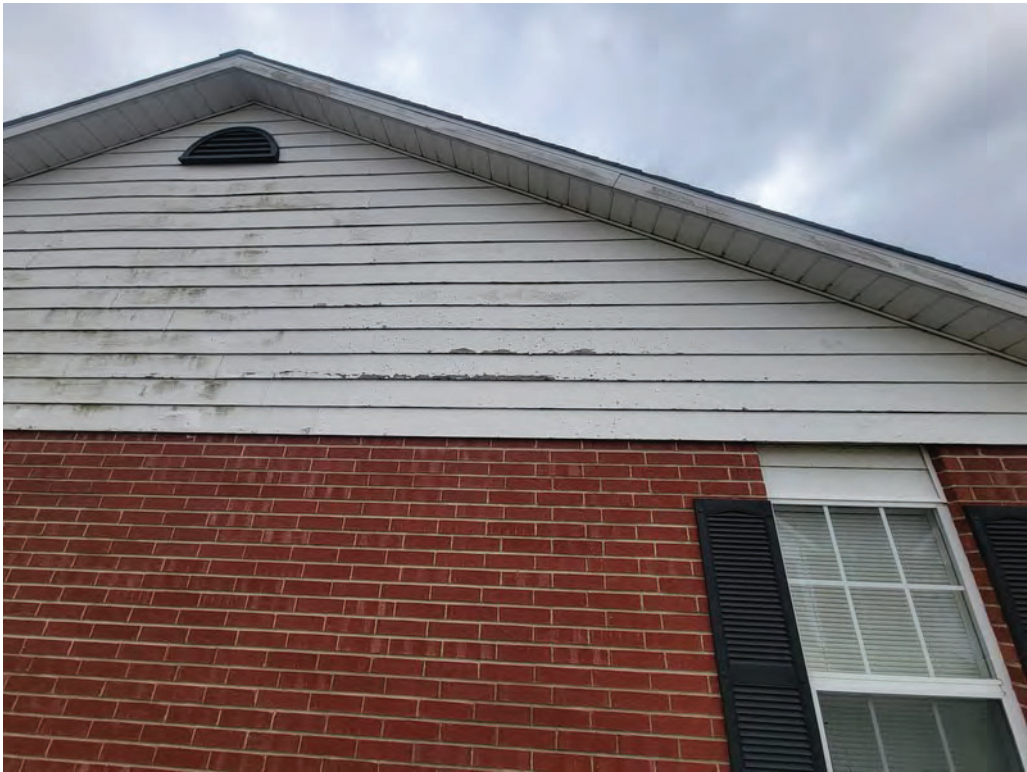
158. Unit building exterior facade
