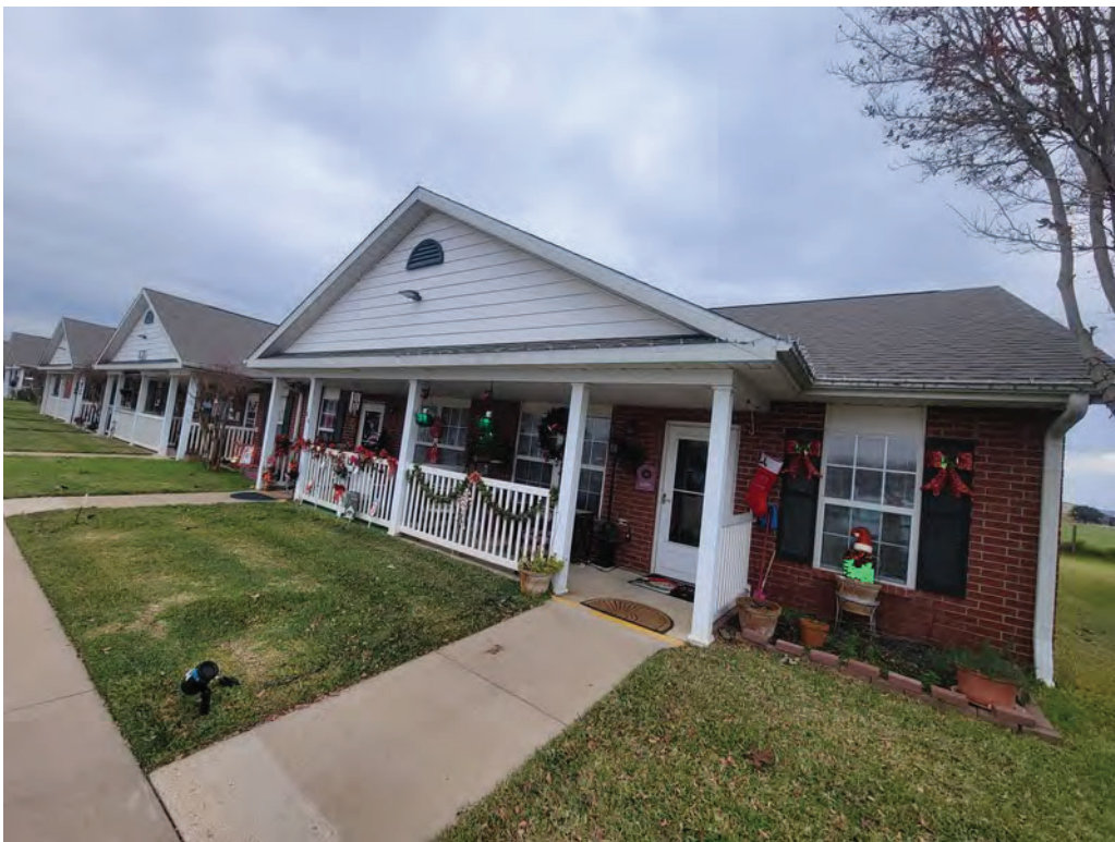
162. Unit building exterior facade
