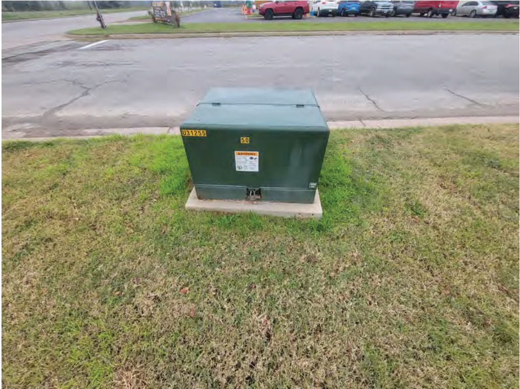
84. Pad-mounted transformer
