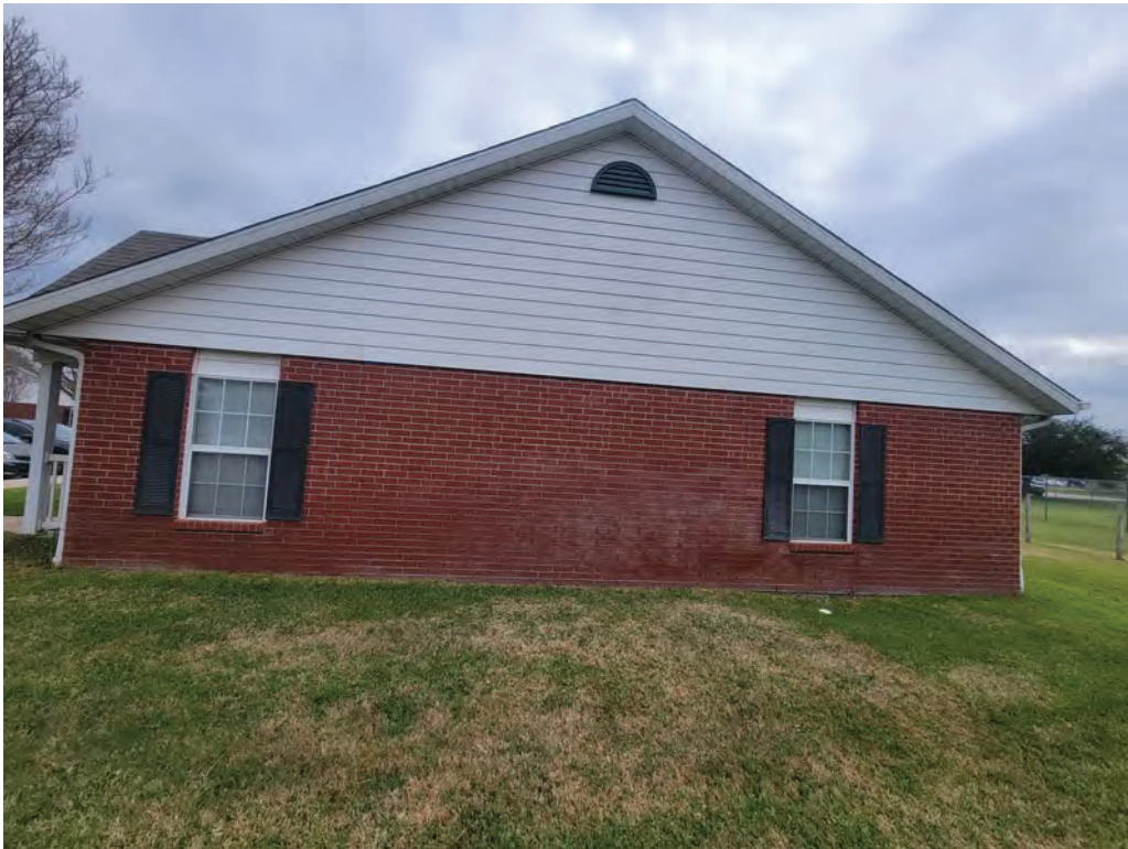
168. Unit building exterior facade
