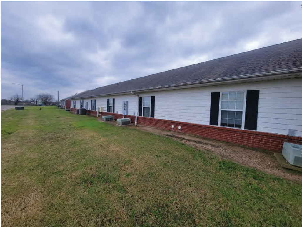
153. Unit building exterior facade
