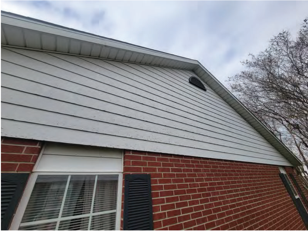
166. Unit building exterior facade
