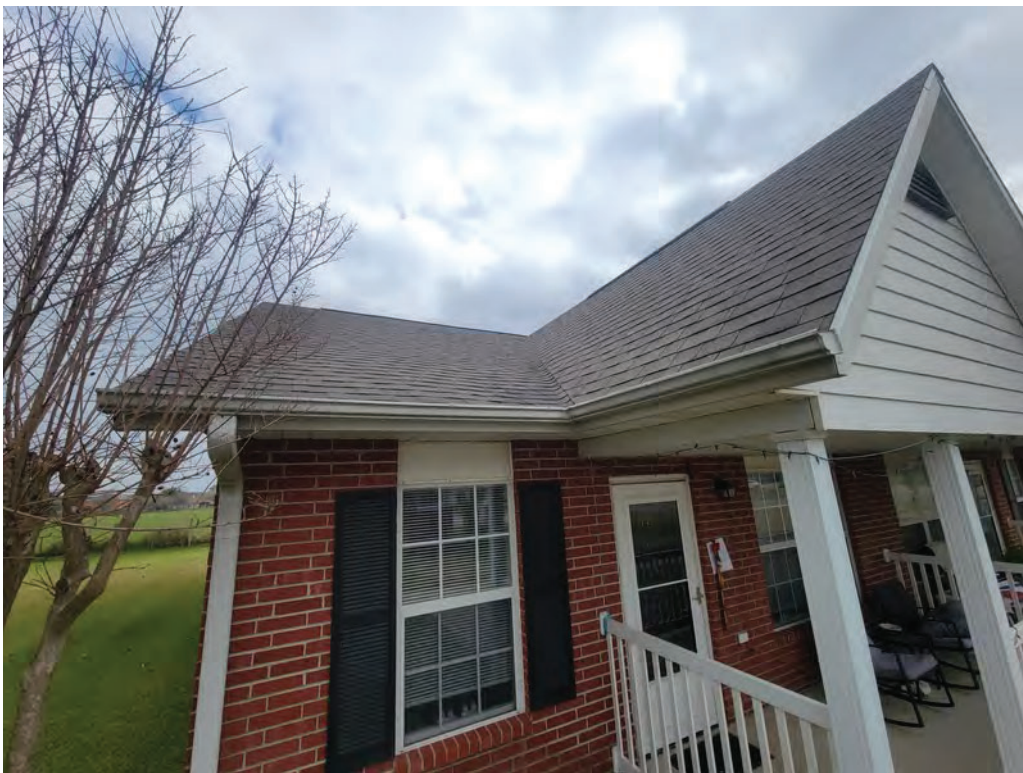
10. Asphalt shingle roofing
