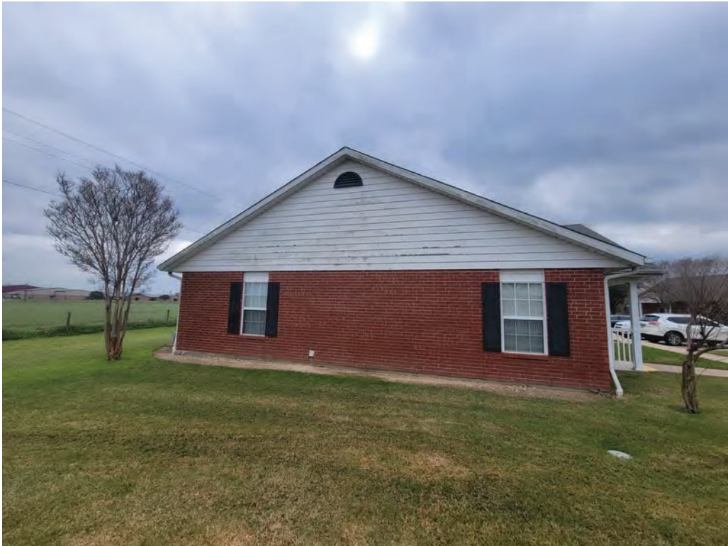
157. Unit building exterior facade
