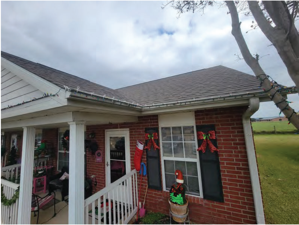
11. Asphalt shingle roofing
