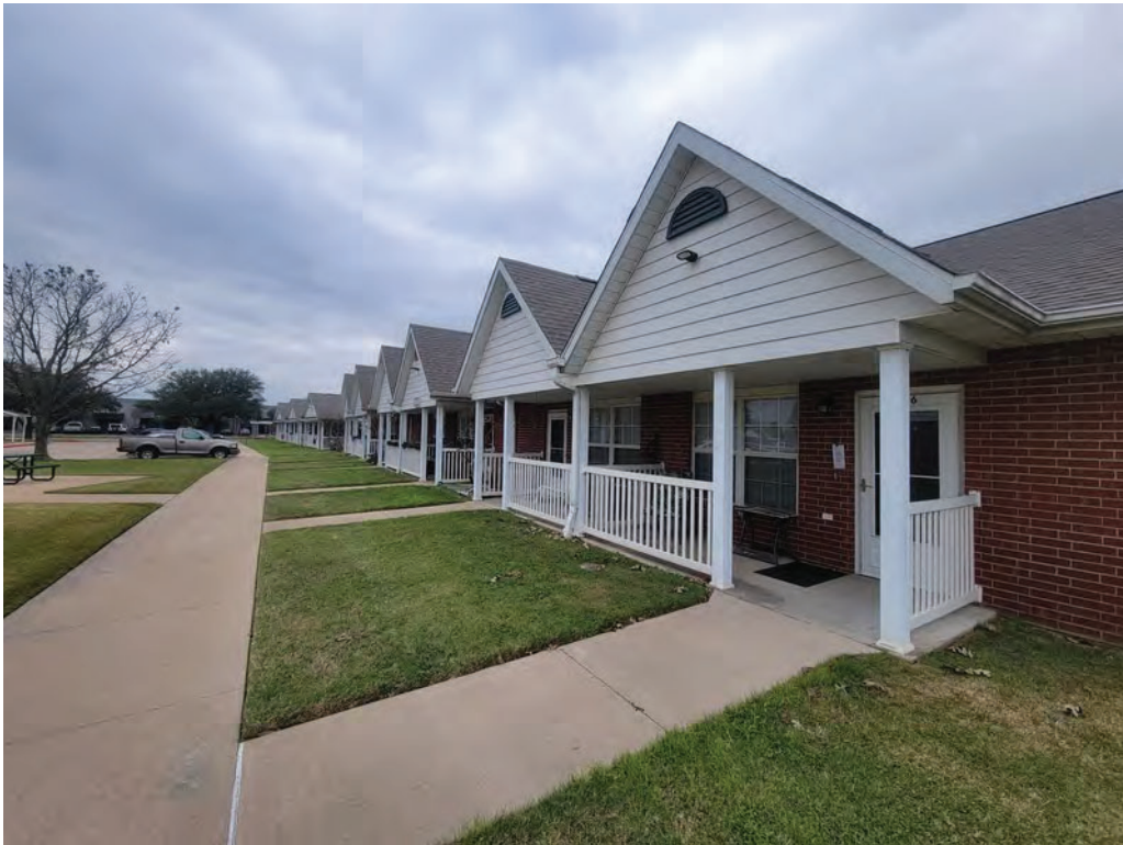
156. Unit building exterior facade
