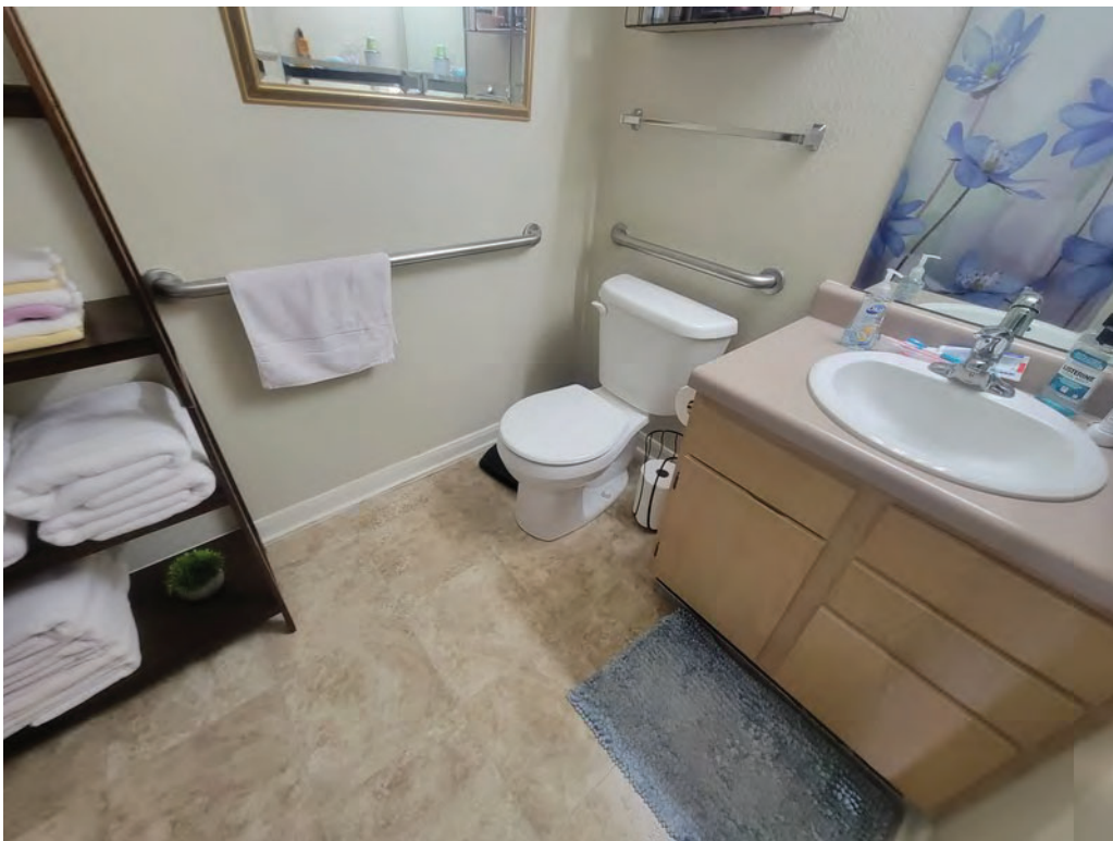
148. Unit ADA bathroom
