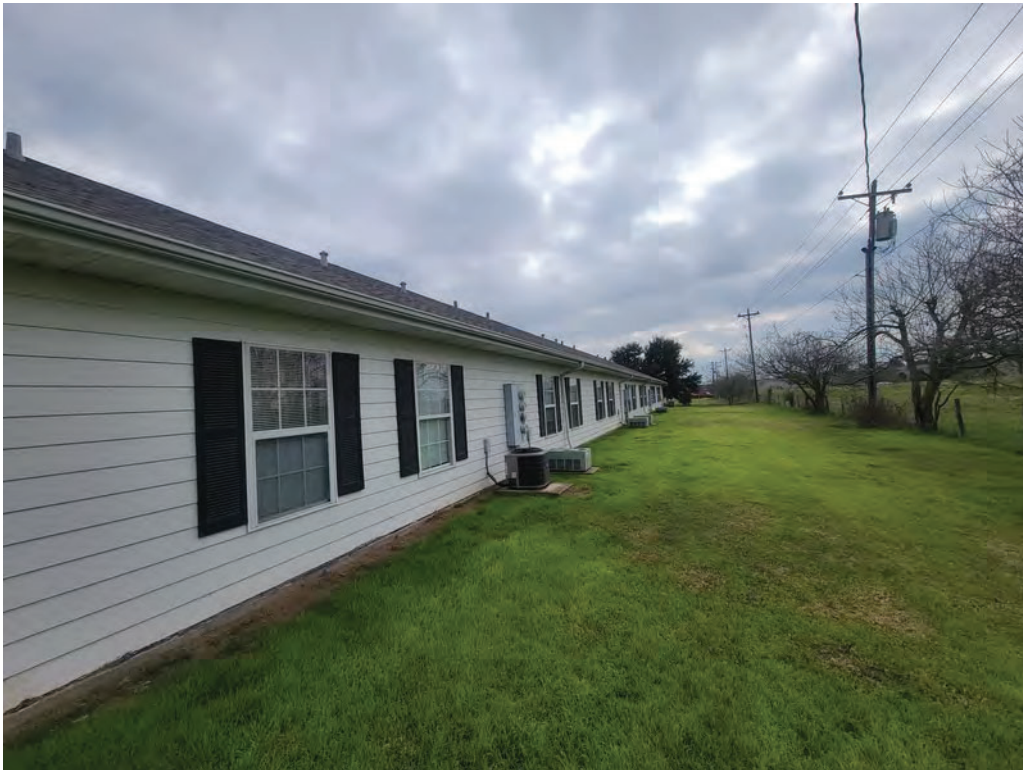
150. Unit building exterior facade
