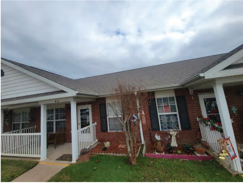
12. Asphalt shingle roofing
