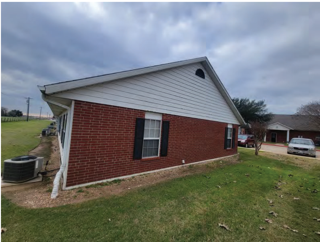
160. Unit building exterior facade
