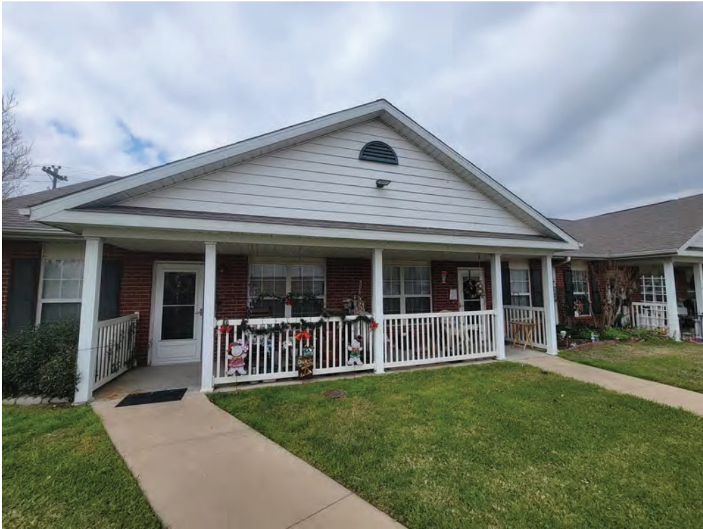
167. Unit building exterior facade
