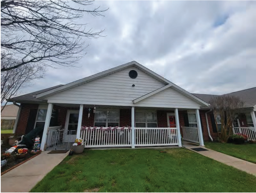
164. Unit building exterior facade
