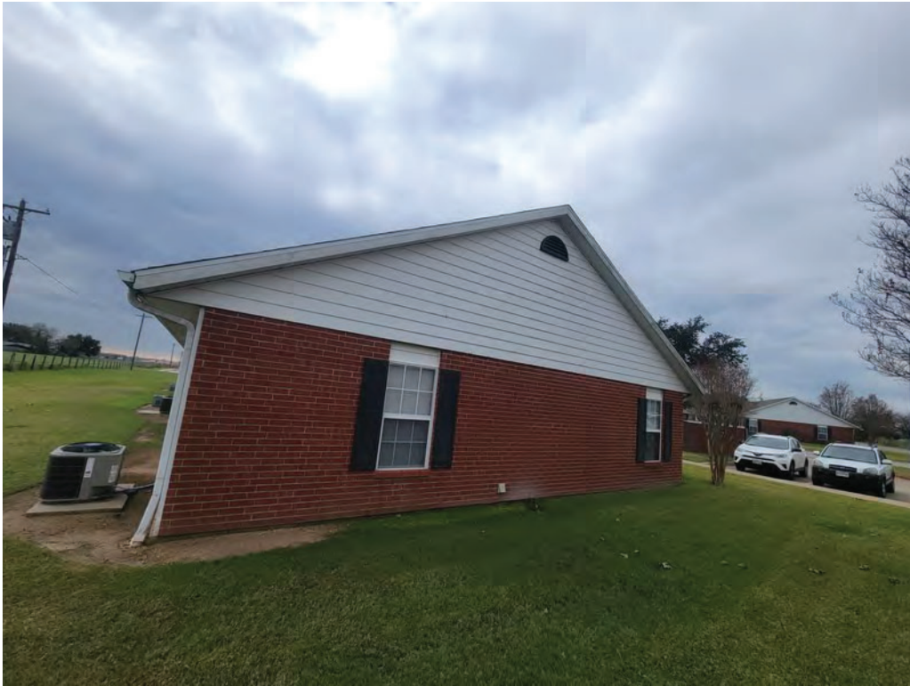
161. Unit building exterior facade
