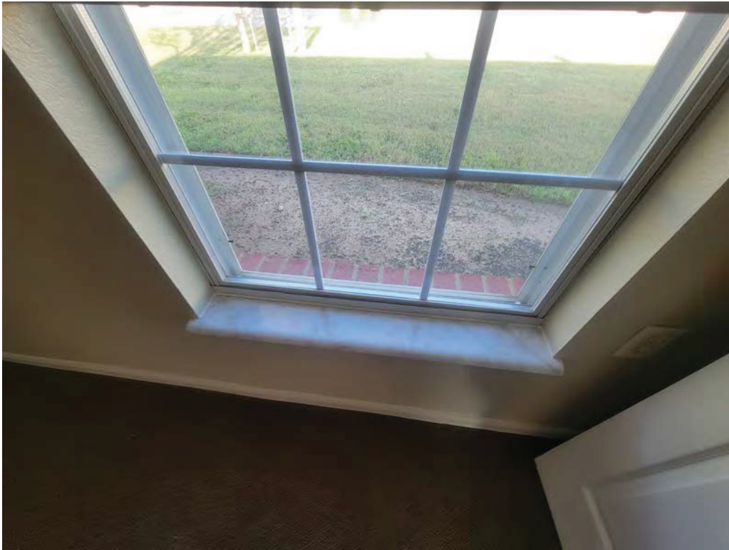
147. Typical window interior view
