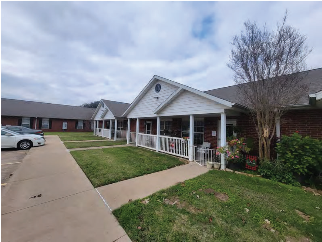
163. Unit building exterior facade
