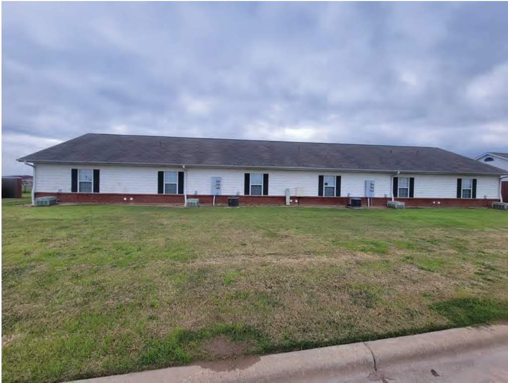
155. Unit building exterior facade
