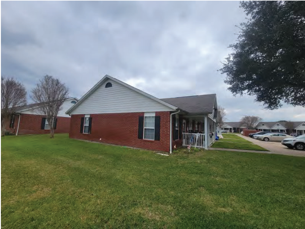
151. Unit building exterior facade
