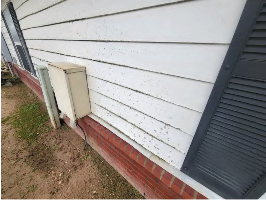
154. Unit building exterior facade
