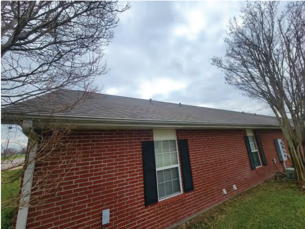
9. Asphalt shingle roofing
