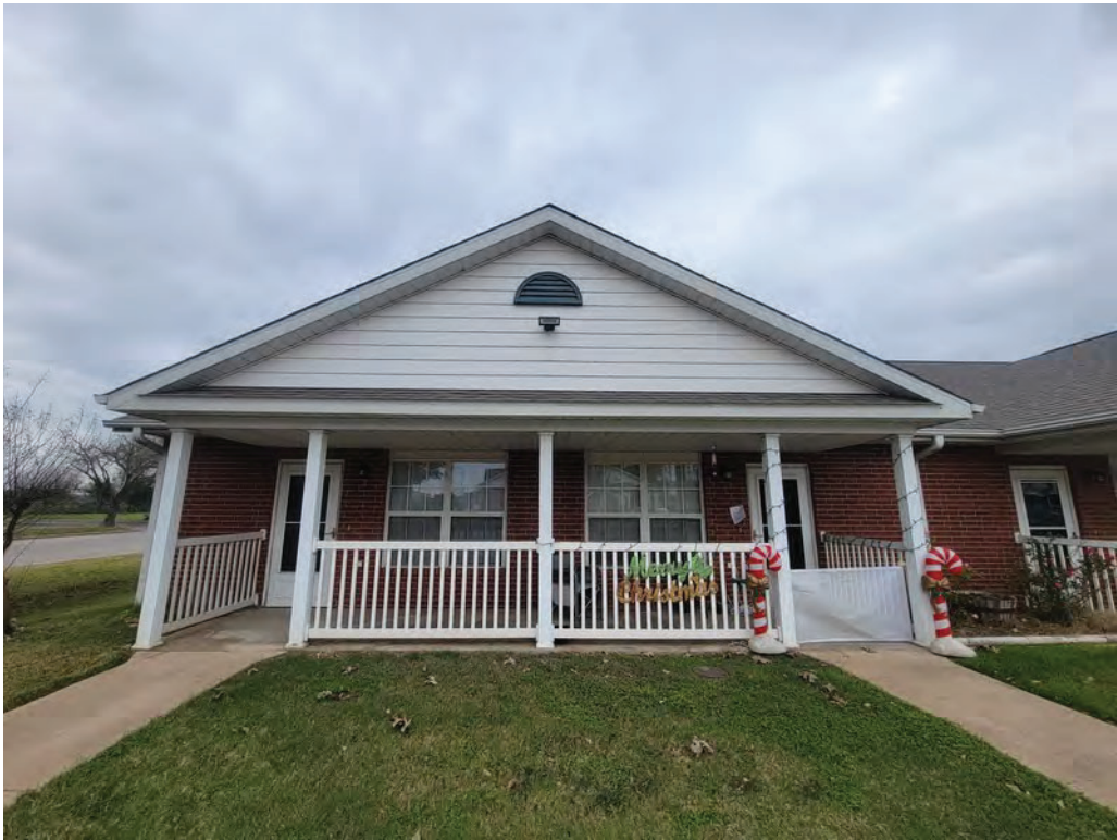
152. Unit building exterior facade
