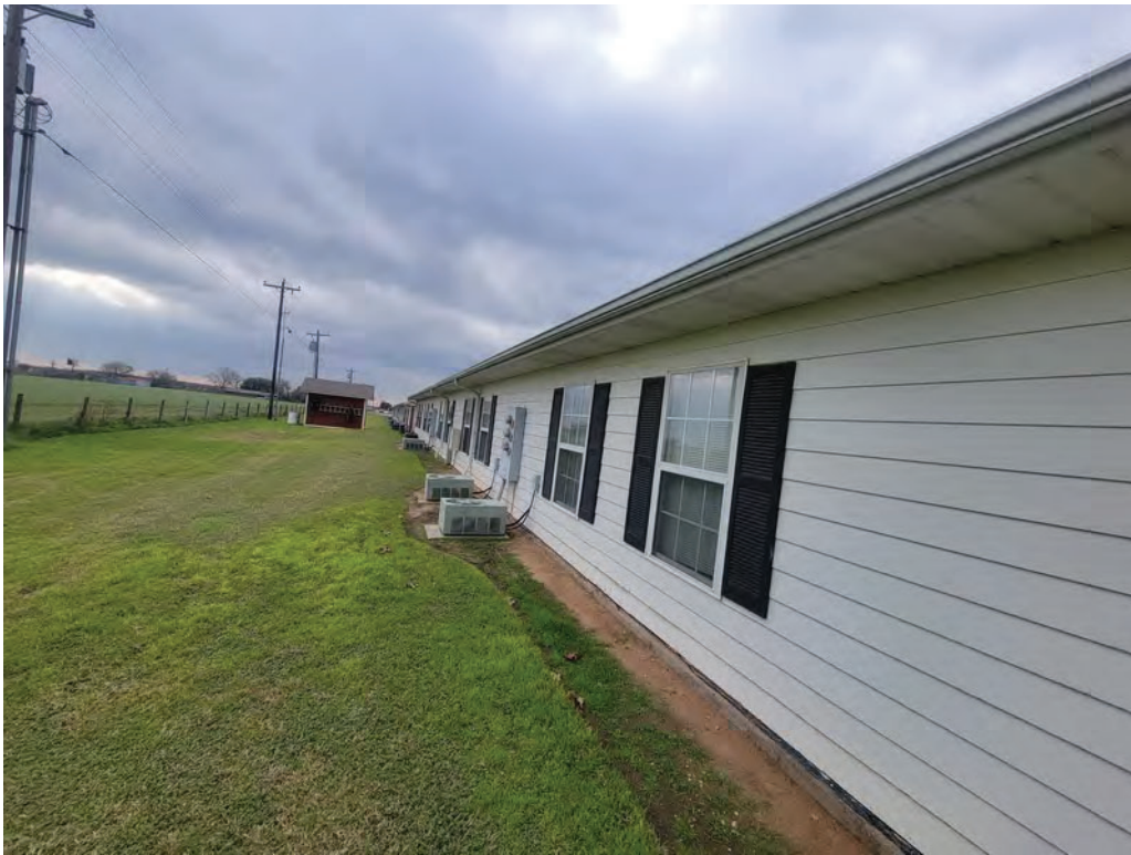
159. Unit building exterior facade
