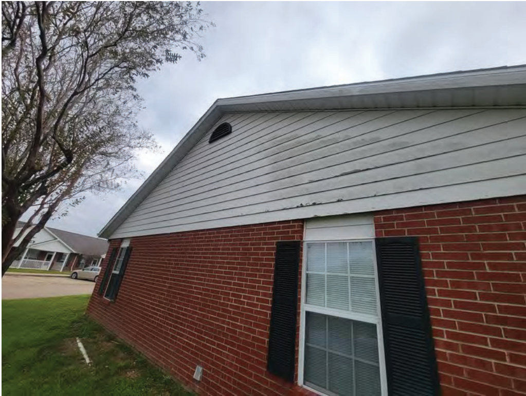
149. Unit building exterior facade
