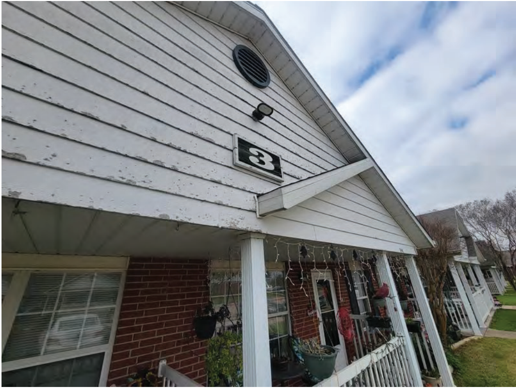
165. Unit building exterior facade
