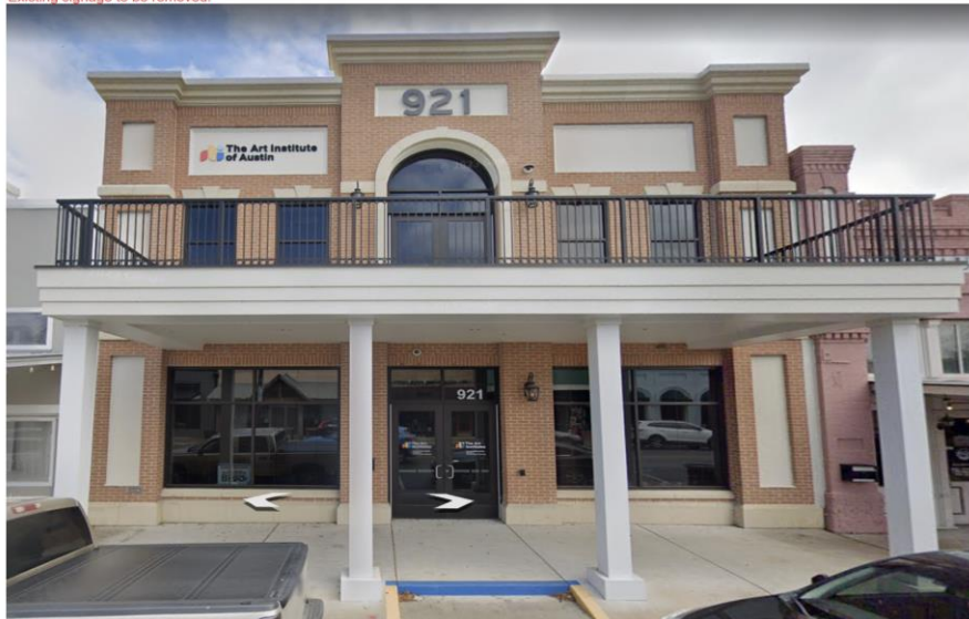
Existing signage to be removed.
