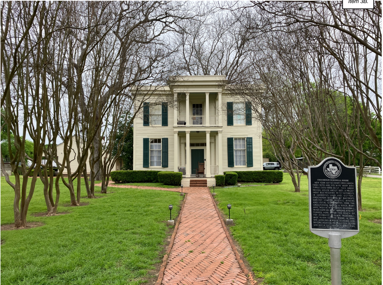
Crocheron House; View looking West from Wilson Street at the front elevation. Photo 2023 GFA
