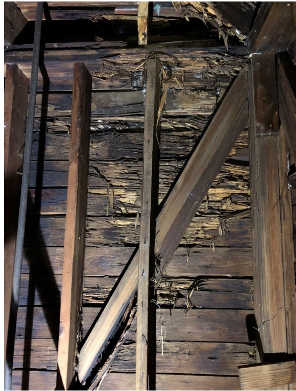
Photo 4: Existing conditions at tower framing
