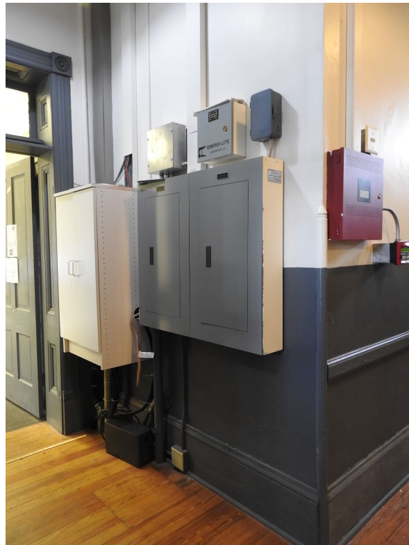
Photo 12: Electrical panels at first floor entry hall to be relocated.
