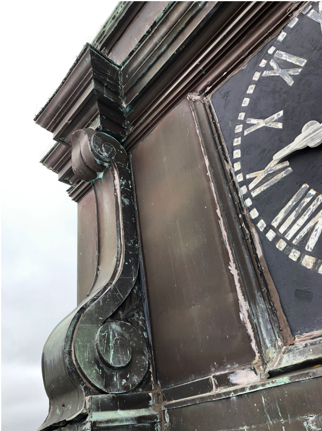
Photo 2: Detail of existing sheet metal cladding and clock face.
