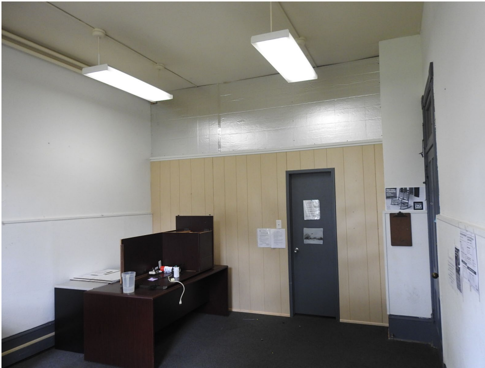
Photo 14: Non-original partitions will be removed, first floor.
