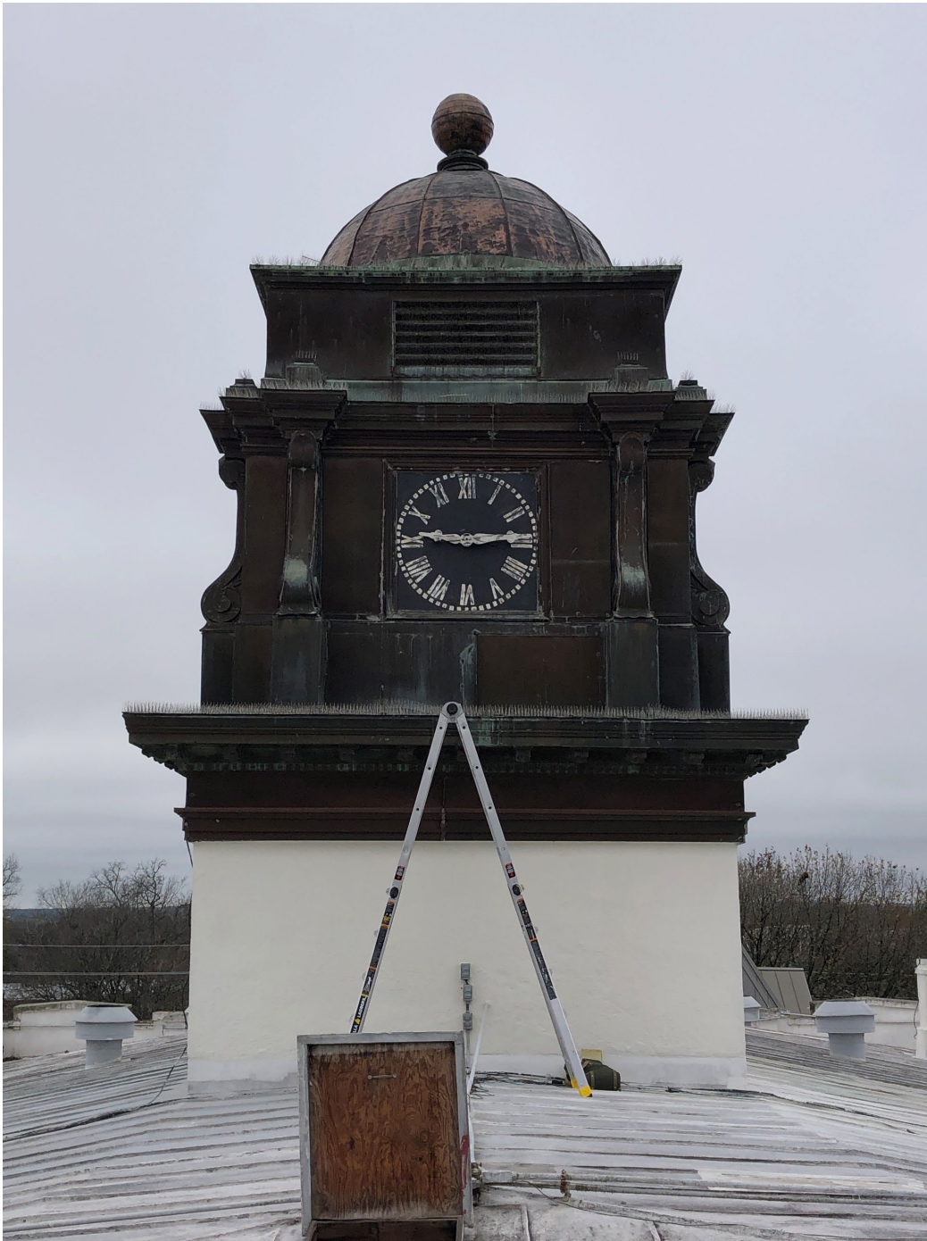
Photo 1: Courthouse tower, existing conditions
