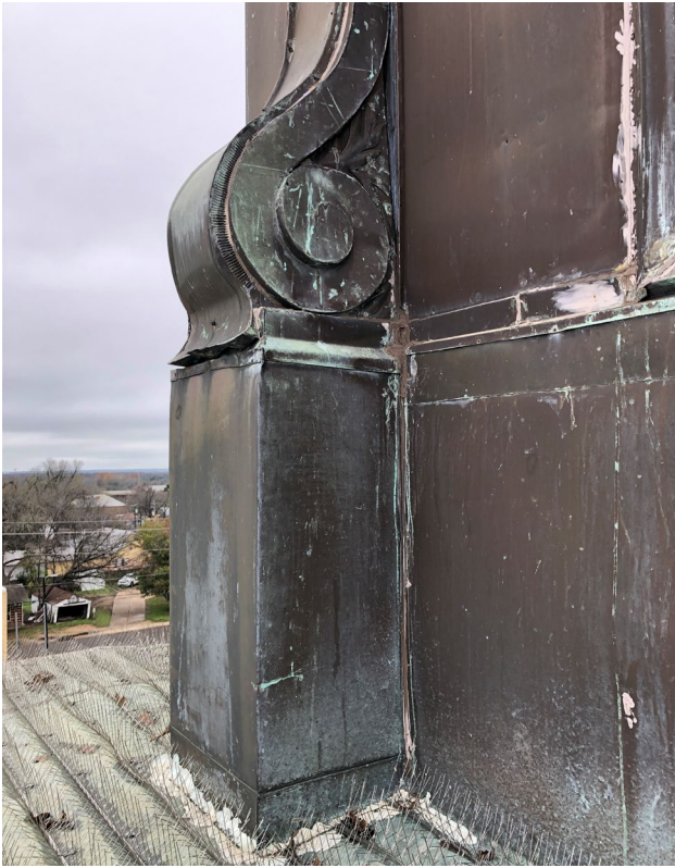
Photo 3: Detail of existing sheet metal cladding
