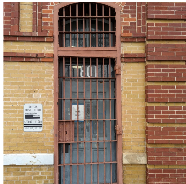
Photo 10: Exterior door and gate to be restored 100%.
