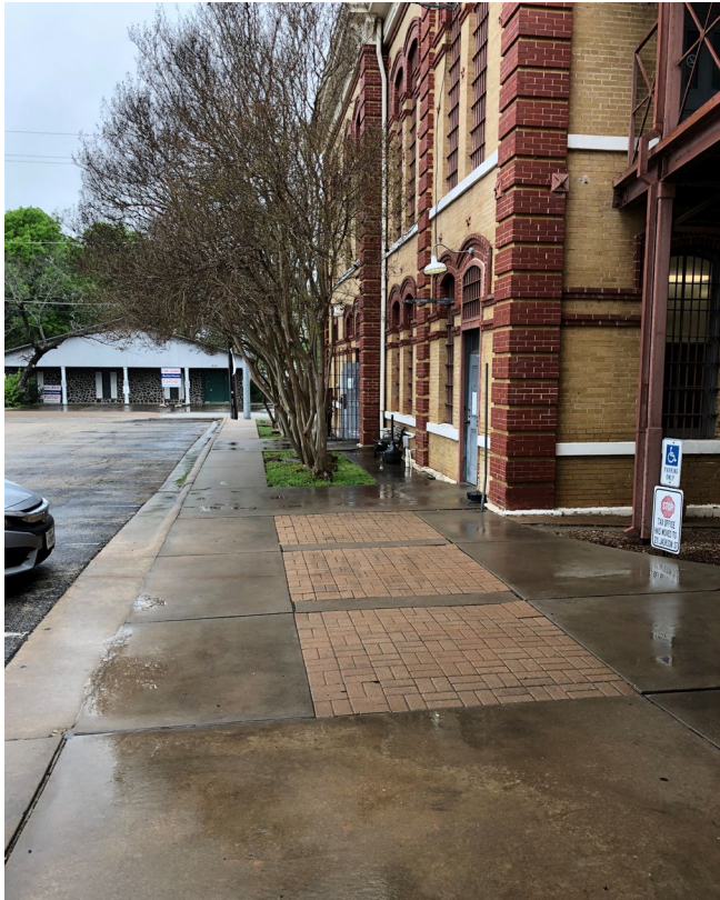
Photo 3: Perimeter of building will receive 2' wide concrete mow strip.
