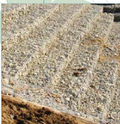
EROSION CONTROL TERRACE BLOCKS / GABIONS
