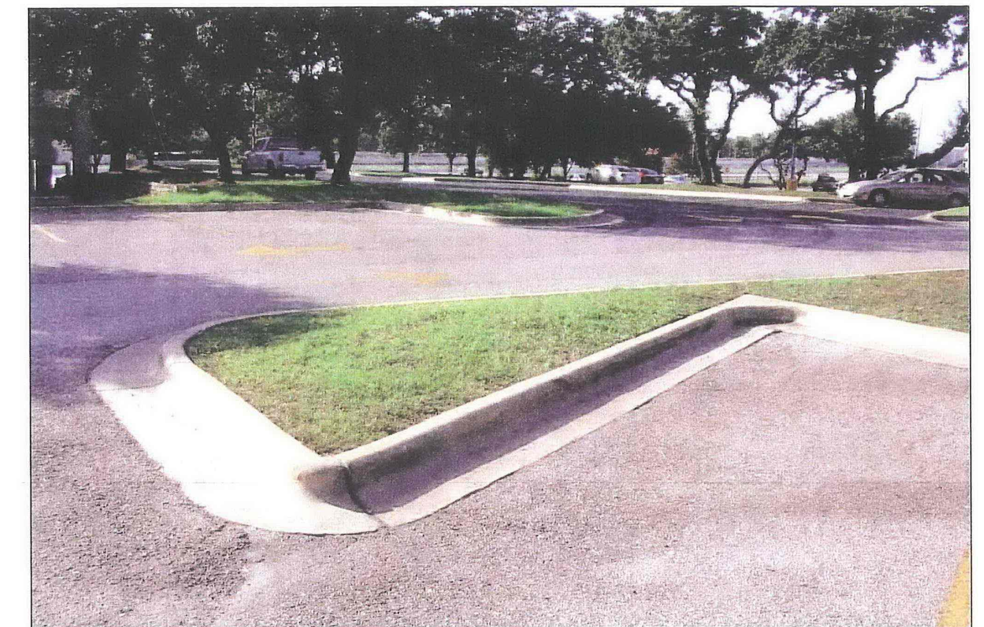
This is an general example of the landscaping in certain end islands and medians.
