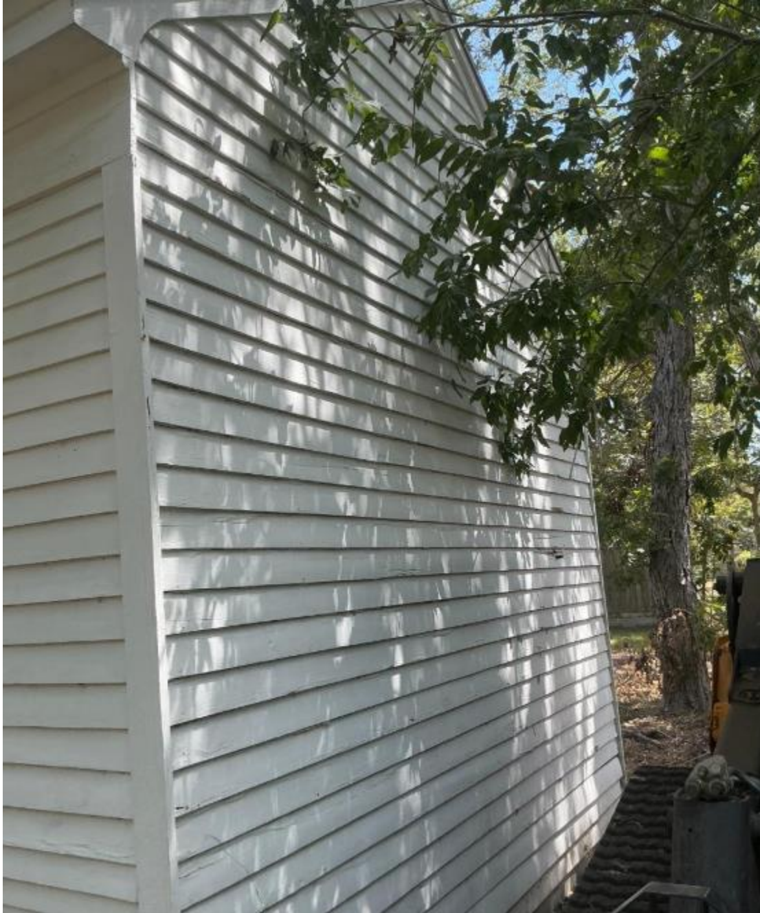
West Elevation – Back view of the outbuilding
