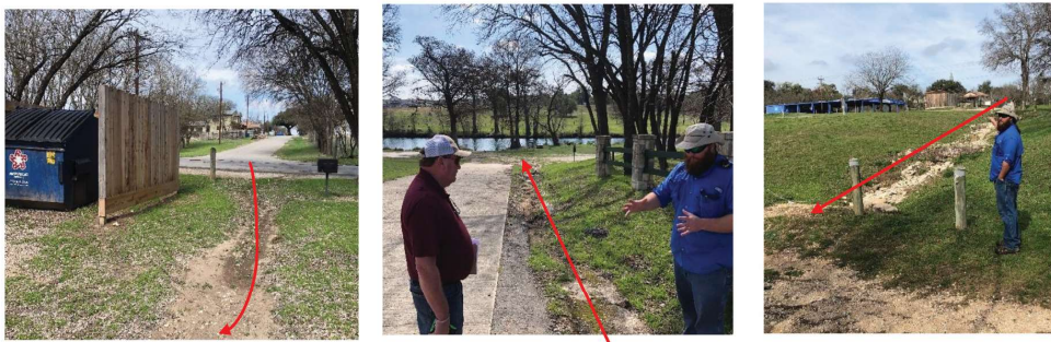
Figure 5: Examples where stormwater runoff is causing erosion from the top of the park down to the river.
