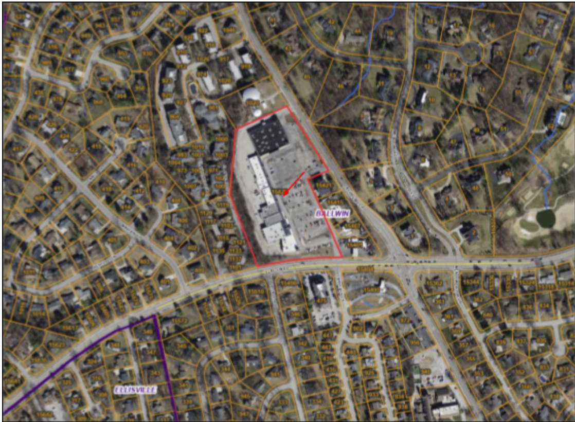
Figure 1 - Aerial view of the site and surrounding properties. The proposed restaurant location is indicated by a red arrow. Source: St Louis County
