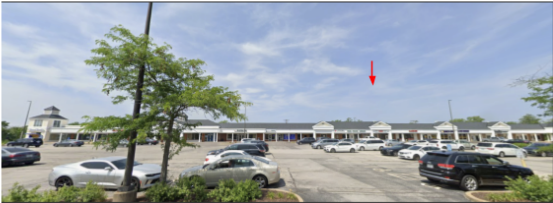
Figure 2 - Street view of the development. The proposed restaurant location is indicated by a red arrow.
