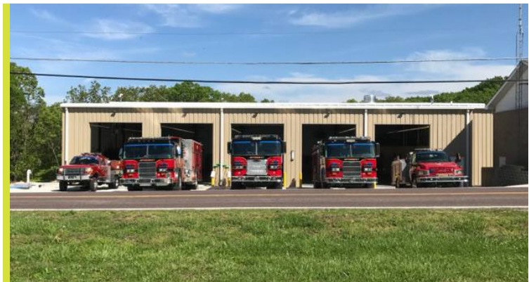
Pre-Engineered Metal Building, Fire Station Apparatus Bays and Support Areas
