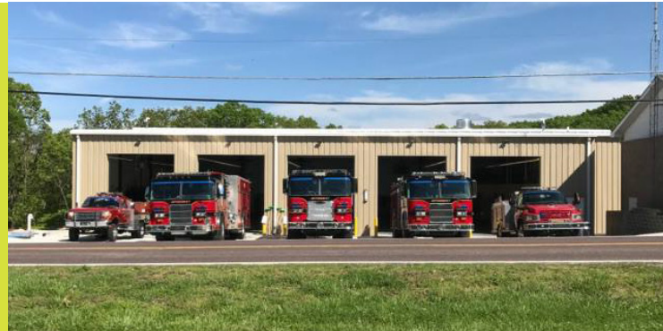
Pre-Engineered Metal Building, Fire Station Apparatus Bays and Support Areas
