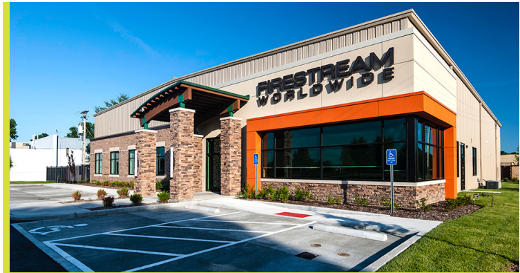
Pre-Engineered Metal Building, Maintenance & Storage
