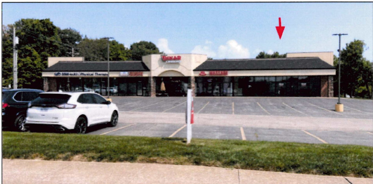
Figure 2 - Street view of the development. The proposed restaurant location is indicated by a red arrow.
