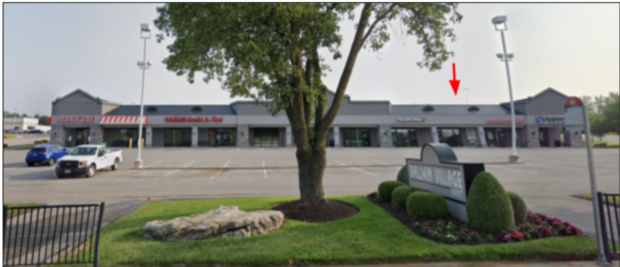
Figure 2 - Street view of the development. The proposed restaurant location is indicated by a red arrow.
