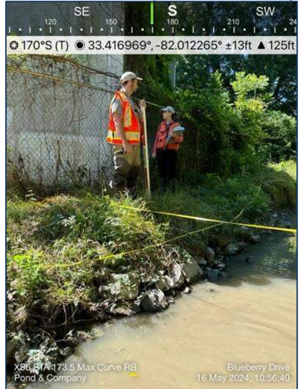
Photograph 8: Looking upstream at right bank; downstream of active erosion adjacent to metal building.
