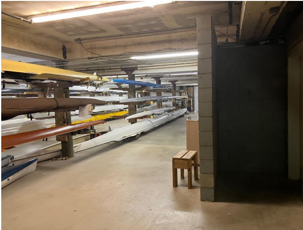
Rowing Club storage, lower level. Note pole construction and associated drywall-covered wood girder framing.
