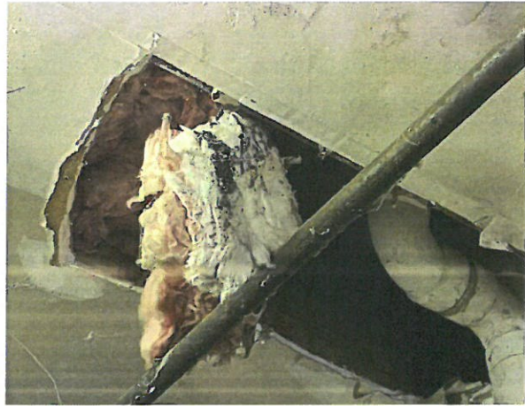
2, Staining Indicative of Mold Colonization on Insulation
