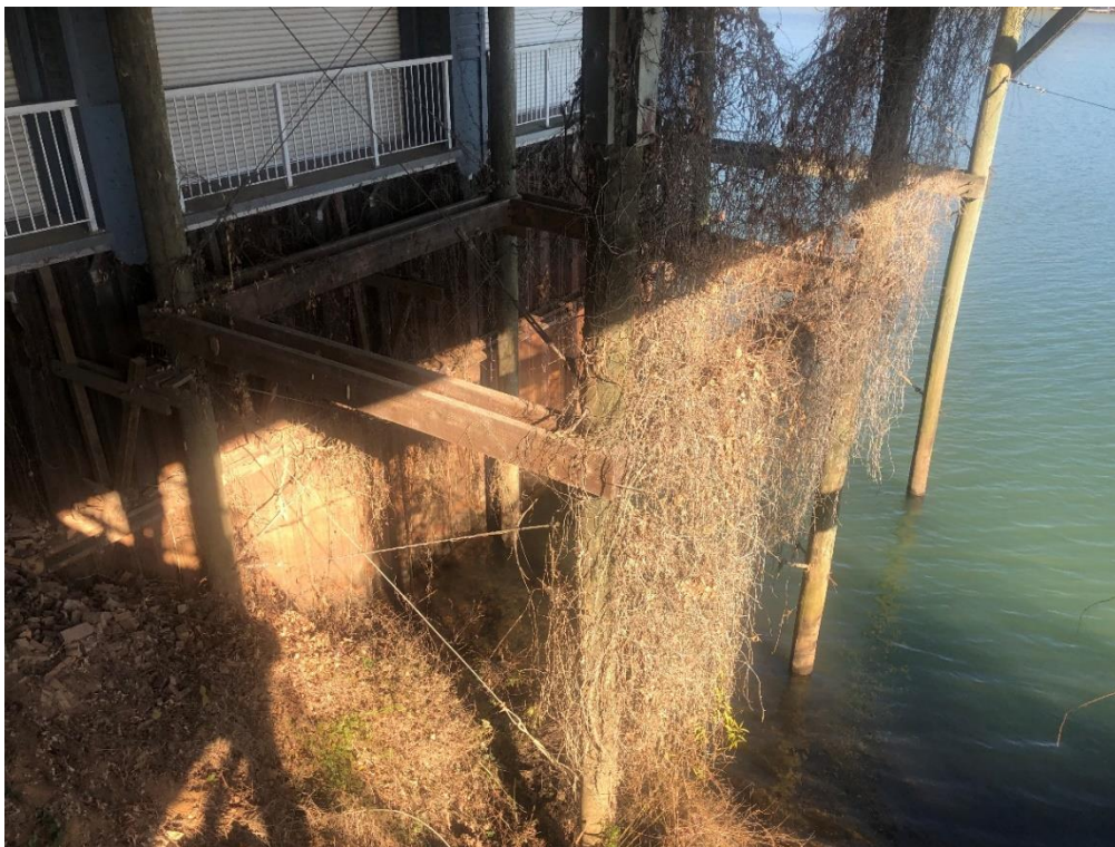
River leg deck pole supports. Some supported on concrete piers others driven into the riverbed.
