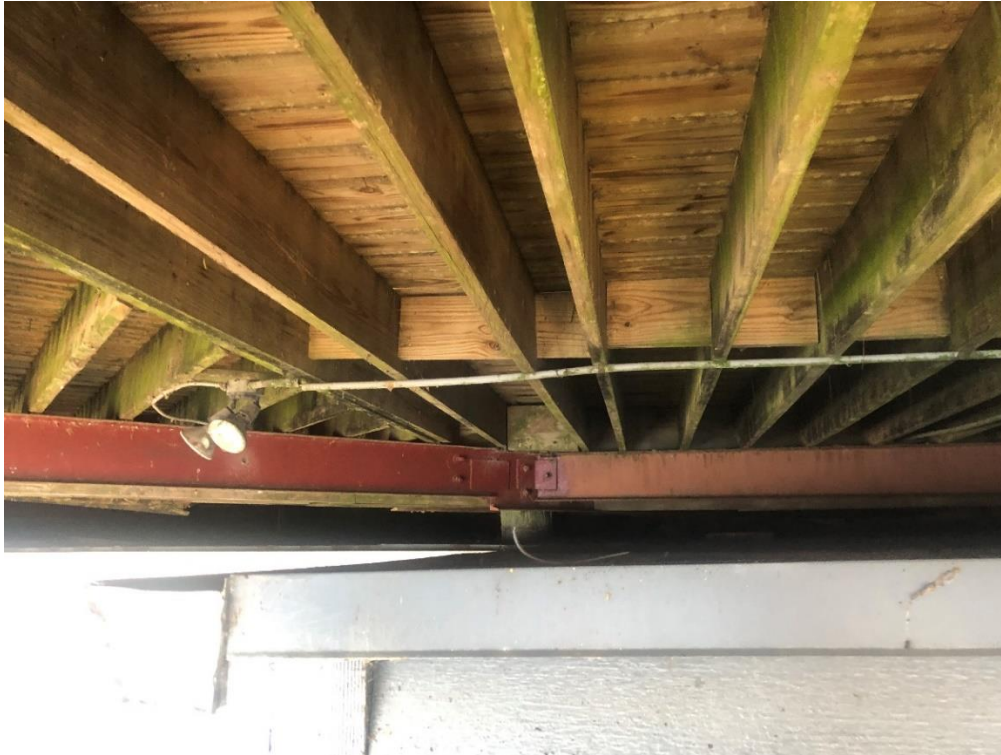
Deck framing above lower enclosure. Note pole support.
