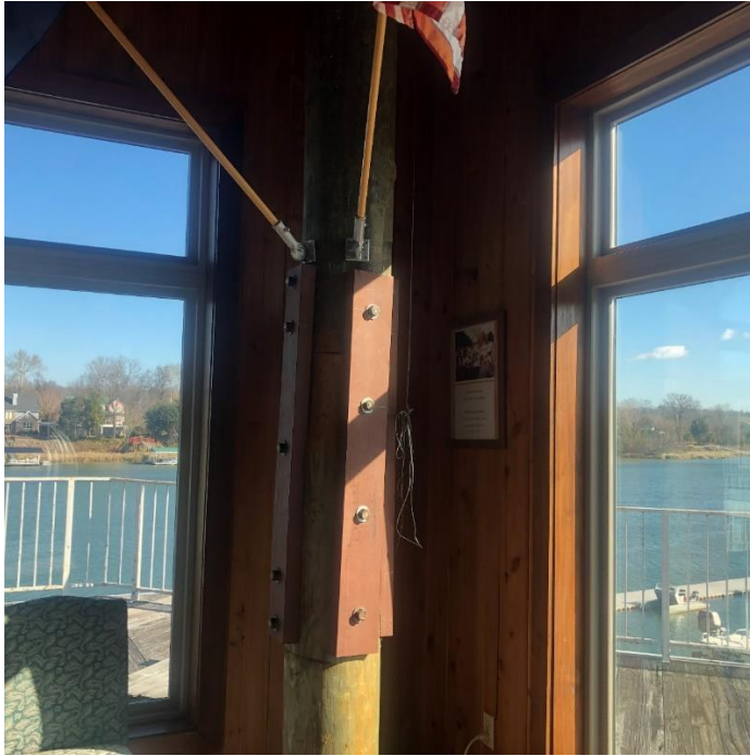
Structural splice at corner pole.
