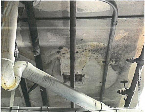
6, Staining Indicative of Mold Colonization Drywall Ceiling
