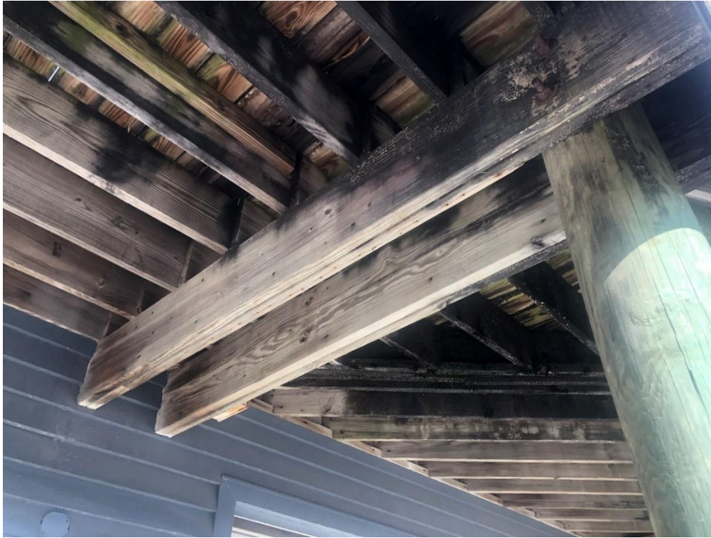
Underside of East deck showing typical poles supported construction
