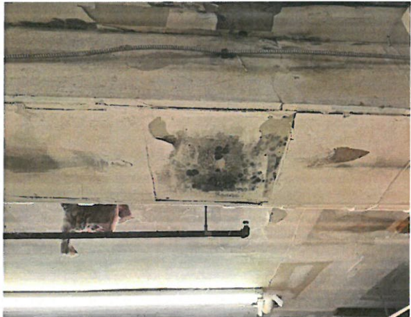
4, Staining Indicative of Mold Colonization Drywall Ceiling
