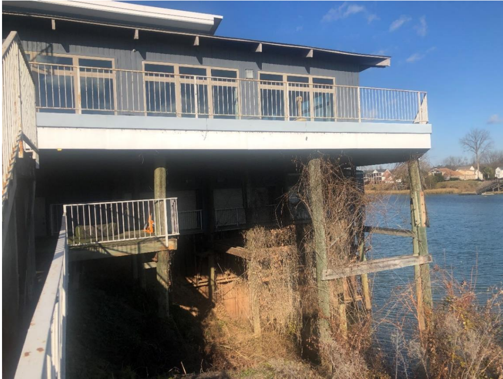
River leg showing sheet pile platform at embankment. Note garage doors with railings around perimeter.
