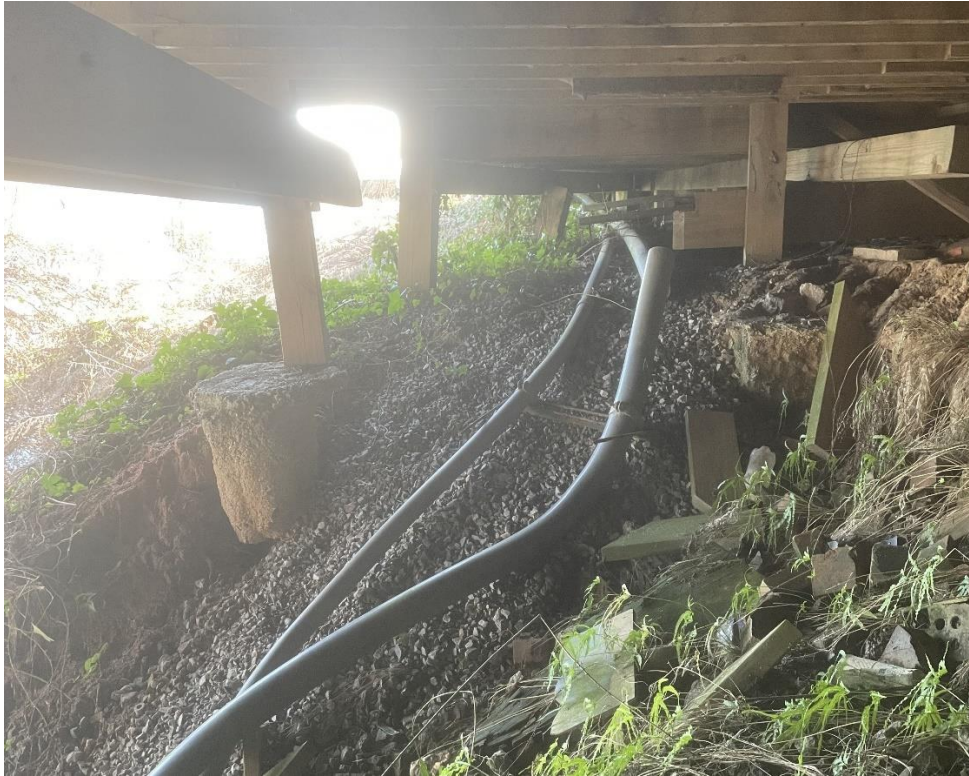
Erosion-compromised (non-pile) deck pier supports.
