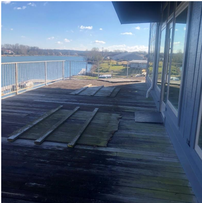
North deck showing previous "repair" attempts.
