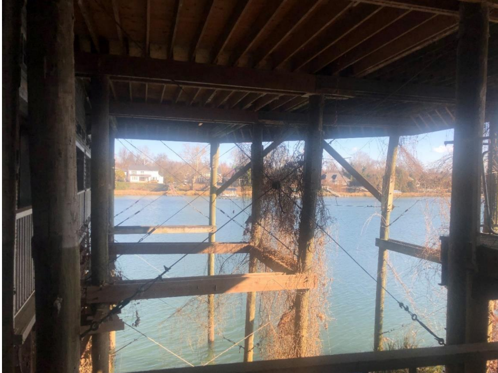
Cable cross bracing at deck support poles.
