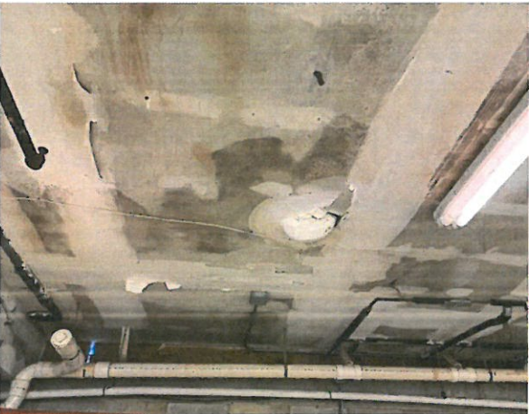
3, Evidence of Water Intrusion and Damage to Drywall
