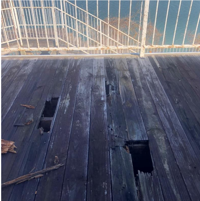
Common existing foot-sized holes in deck.
