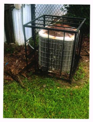
Photo 14. Evidence that HVAC has been submerged.
