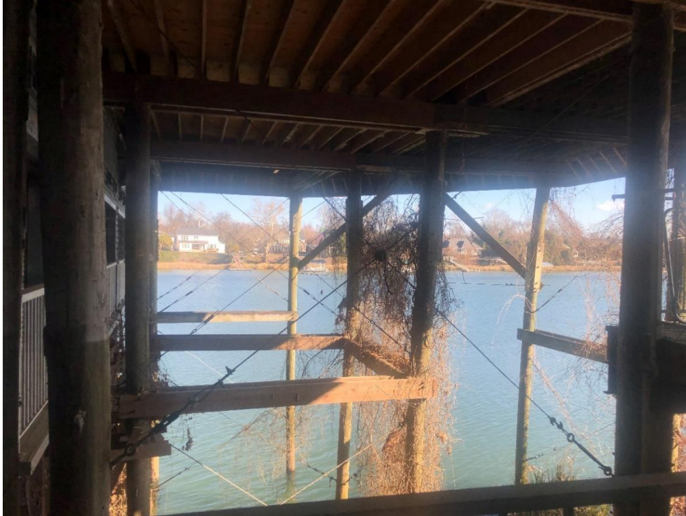
Cable cross bracing at deck support poles.
