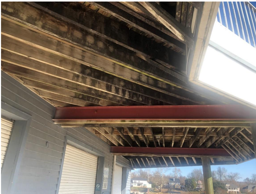
Steel reinforcement of deck girders. Note bad condition of framing beyond the protective building eaves of roof above deck.
