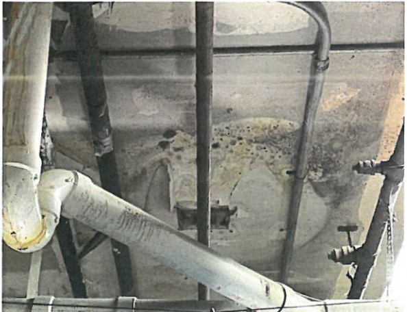
6, Staining Indicative of Mold Colonization Drywall Ceiling
