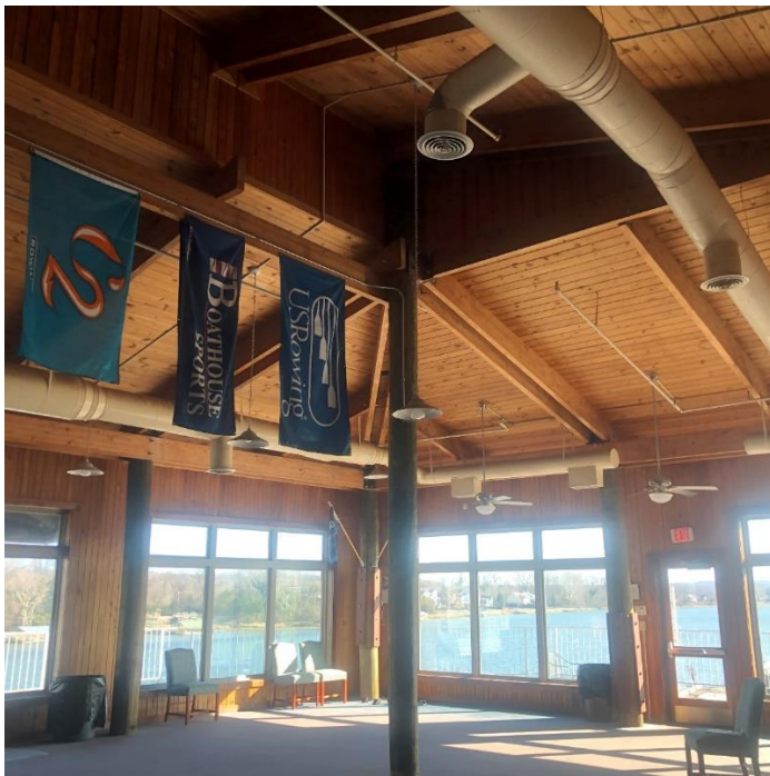
Embankment leg bar area showing typical pole and framing construction.
