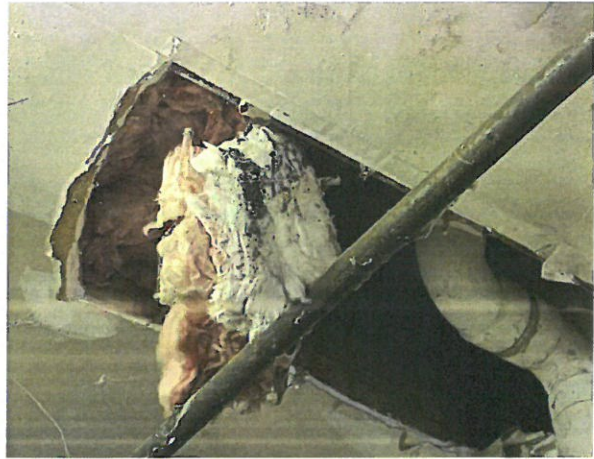
2, Staining Indicative of Mold Colonization on Insulation
