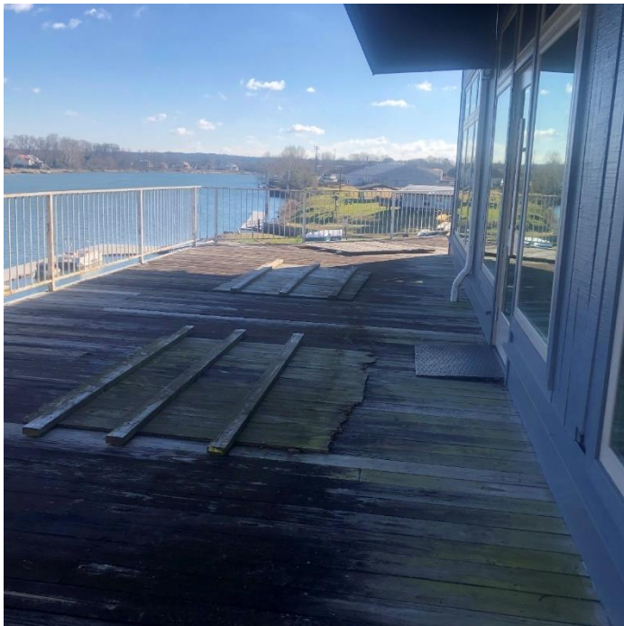
North deck showing previous “repair” attempts.
