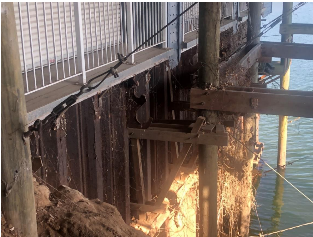
Condition of sheet pile platform and tie-back supports.
