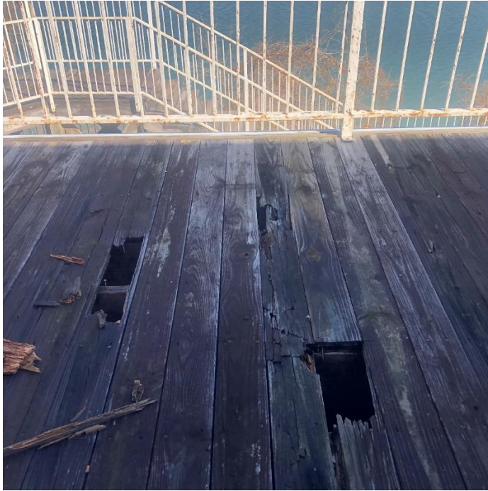
Common existing foot-sized holes in deck.
