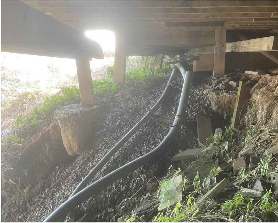
Erosion-compromised (non-pile) deck pier supports.
