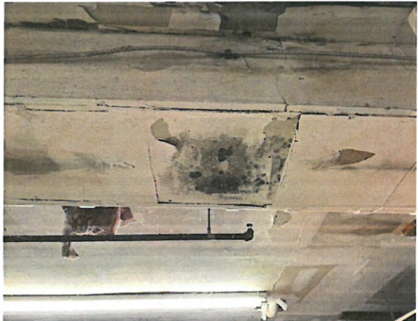
4, Staining Indicative of Mold Colonization Drywall Ceiling
