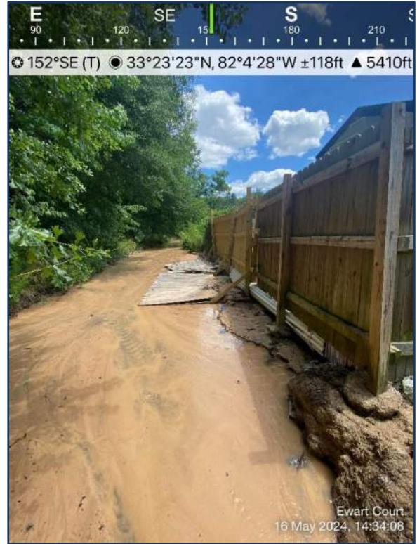
Photograph 2: 2010 Ewart Court, looking upstream at the left bank adjacent to the failing fence line.
