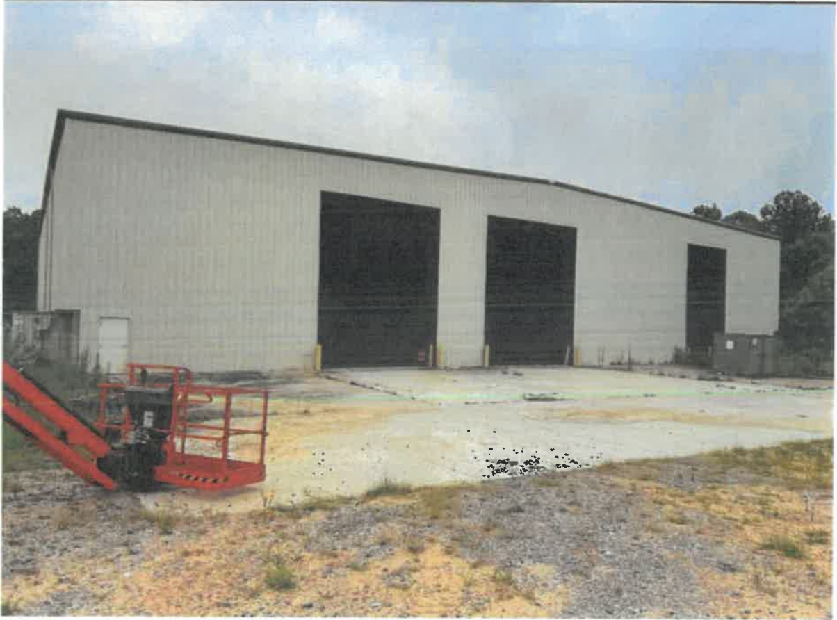
Photo 2: Front of existing Transfer Station Building
