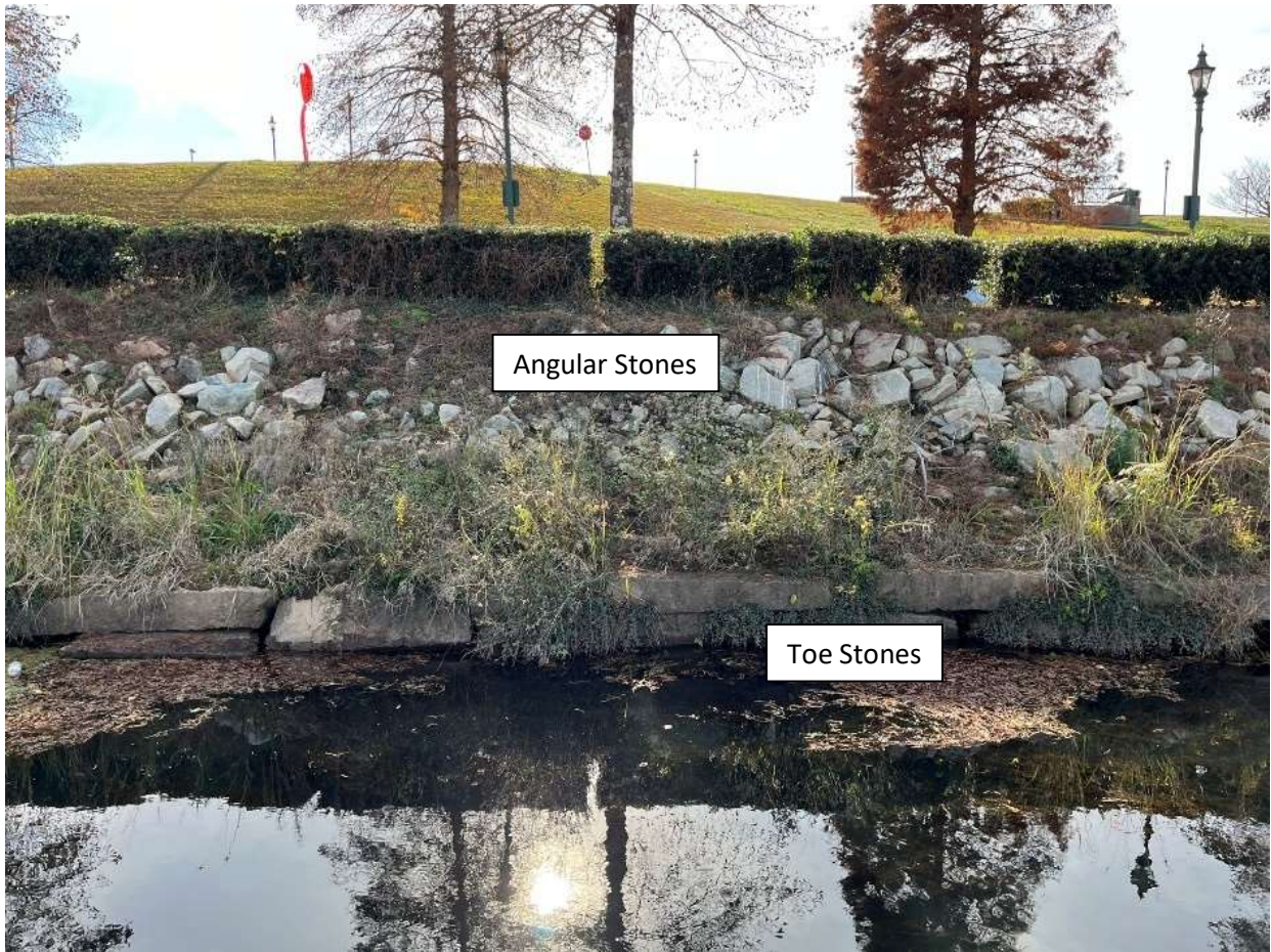
Photo 29 - Typical sloped rock revetment condition (front view)
