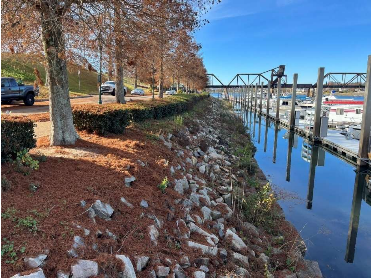
Photo 30 - Typical sloped rock revetment condition (side view)
