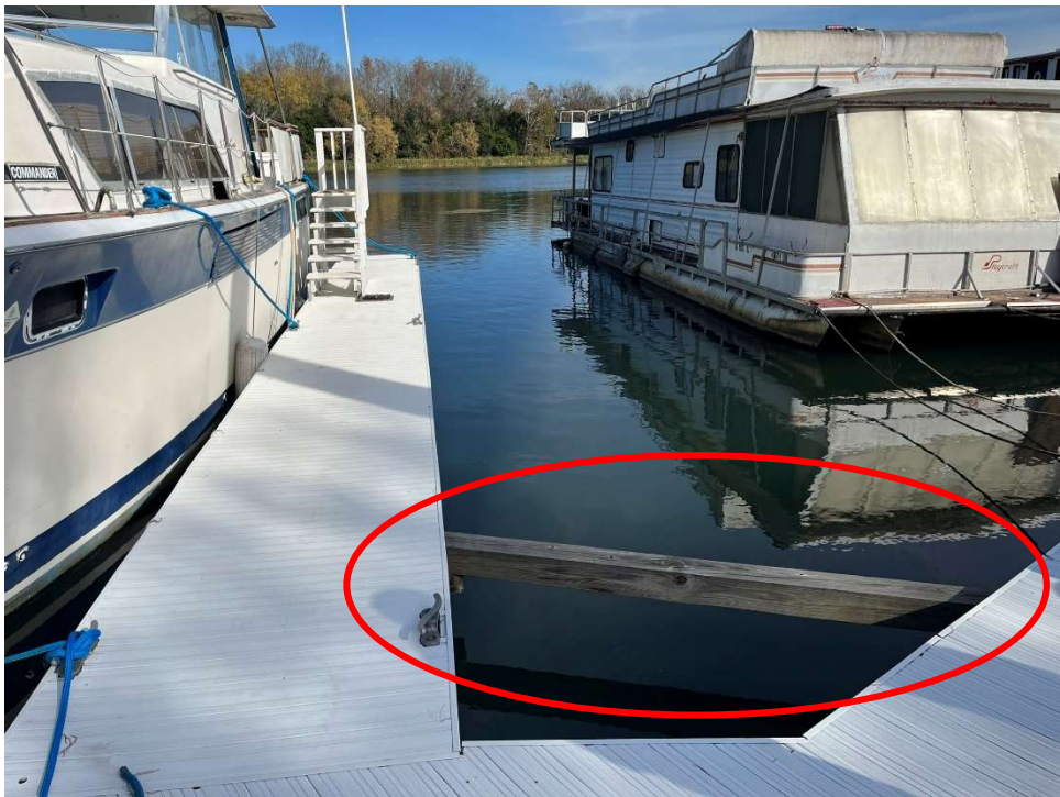
Photo 2 - Typical supplemental timber angle bracing
