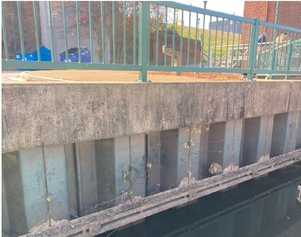
Photo 33 - Steel sheet pile wall typical condition
