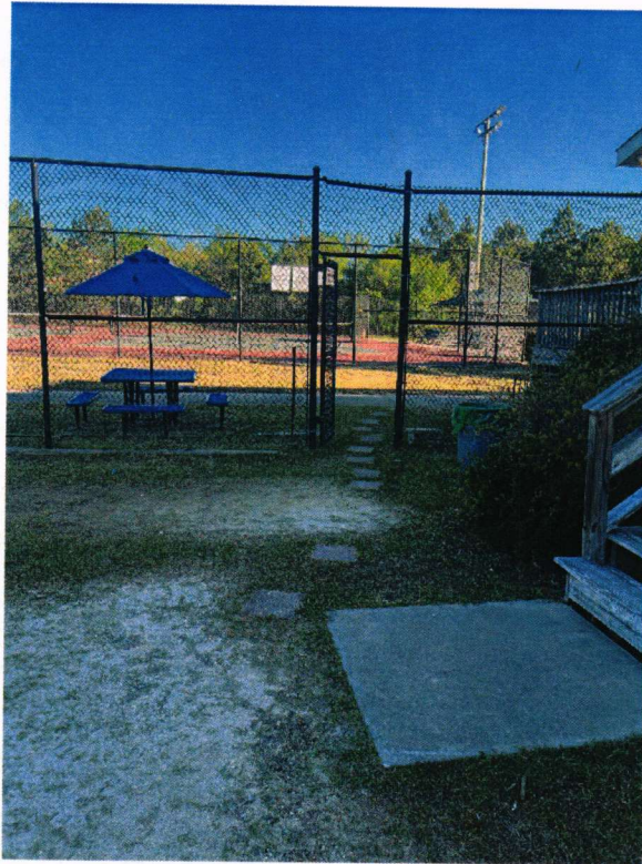
Photo 15. Unstable pathway and narrow gate hinder wheelchair access.
