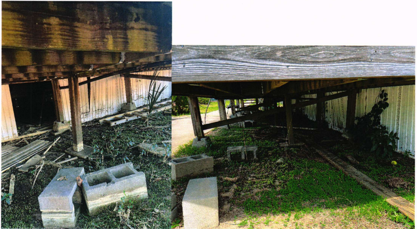
Photos 6, 7, 8, and 9. Unstable support columns.
