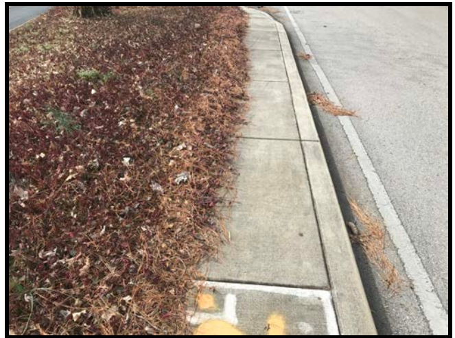
Helen Street- Typical Obstruction Due to Overgrowth
