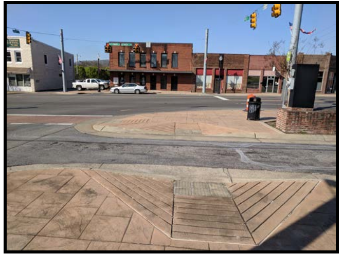
Main St. and HWY 49/Frey St. Excessive Flare Grades, Courthouse Entrance Drive
