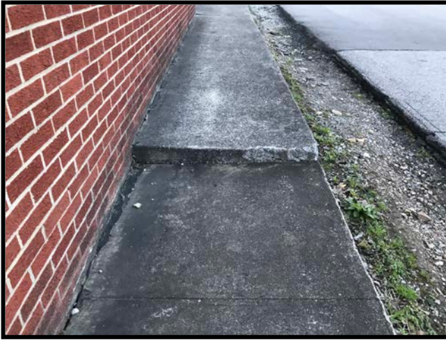
North Vine Street- Changes of Level, Step-ups
