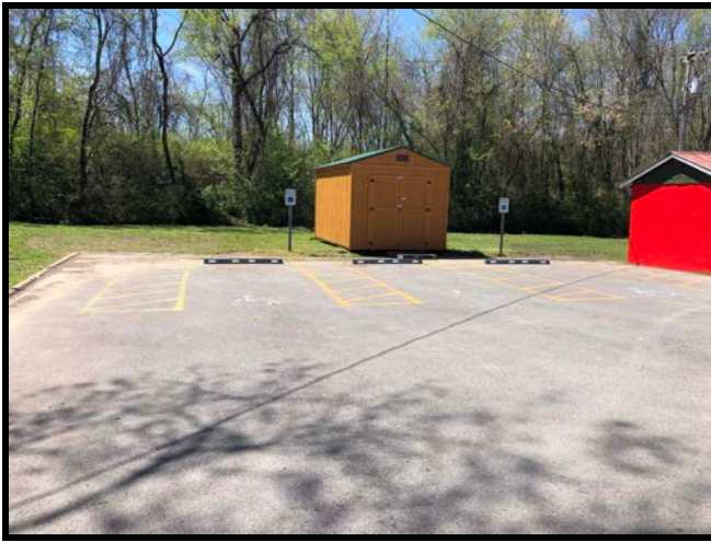
J.W. Johns Jr. Access Aisle & Signage Non-Compliant
