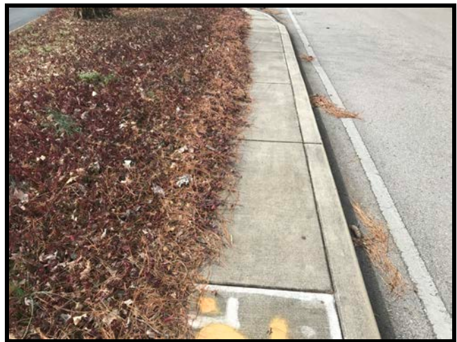
Helen Street- Typical Obstruction Due to Overgrowth
