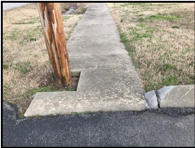
Little Marrowbone Rd. Utility Pole Obstruction
