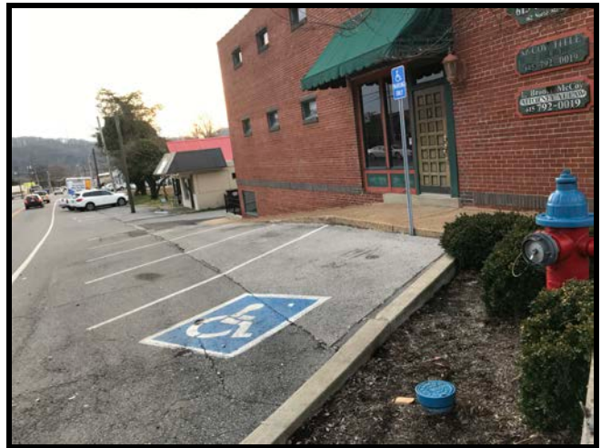
Cumberland Street-On Street Parking No Accessible Aisle or Ramp from Space
