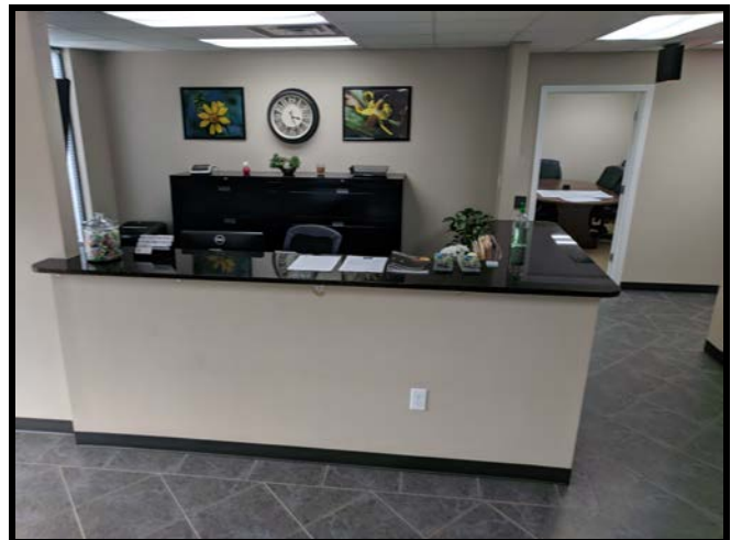
Parks/PW Dept. Service Counter Too High
