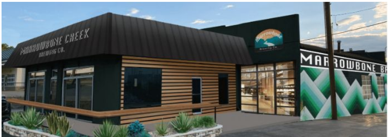
The proposed signage changes to the building. The sign on the north side wall will be approximately 60ft x 3ft with wall color behind the letters. This will accompany a mural below. The sign above the door on the right can be removed if two wall signs will not be permitted.
