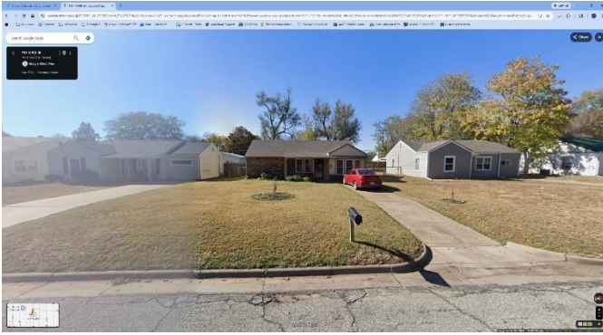
The subject property-Google Streetview October 2024
