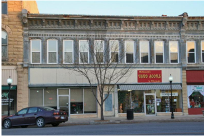
Eagle Block. 312-314 S Summit. Front/west facade. 12-11-2017. B. Spencer
