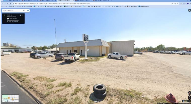
Looking across the Madison Ave to the South. L.G. Pike Construction. Google Streetview from September 2023.
