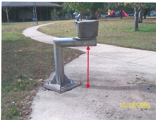
This drinking fountain does not have adequate knee clearance.
