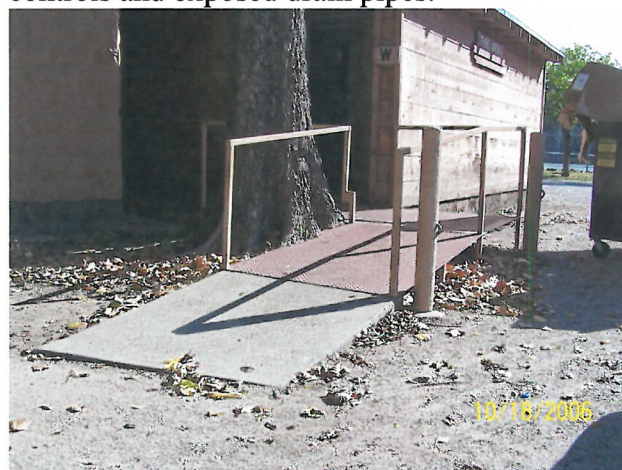
This ramp at the women's restroom is too steep, lacks adequate handrails and edge protection.
