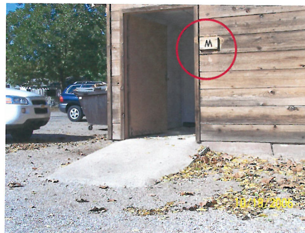
This ramp at the men's restroom is too steep, lacks edge protection, handrails and slopes to the doorway. The sign is mounted too high and is not in an accessible format.
