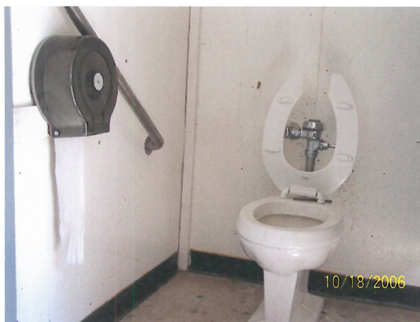
Toilet stalls are too narrow and have improper grab placements and lack bars on rear walls.
