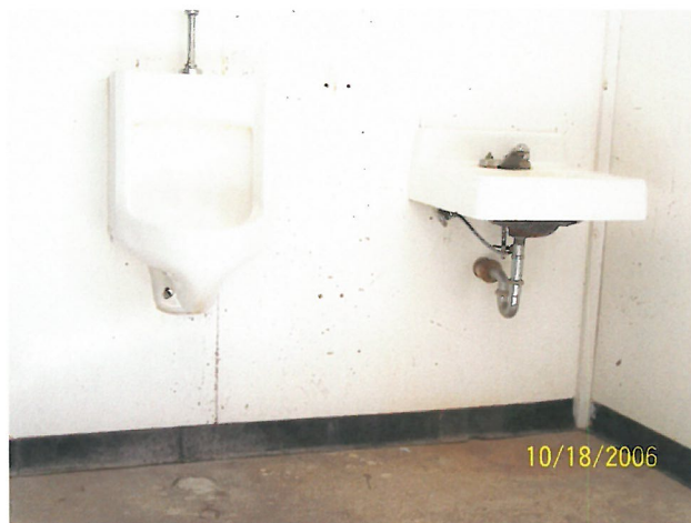
There is enough wall space in the men's restroom to widen the toilet stall. The urinal rim is too high and the lavatory has round faucet controls and exposed drain pipes.
