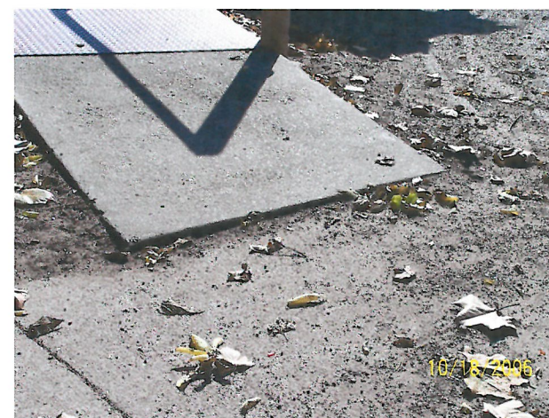
The women's restroom ramp has an excessive threshold.
