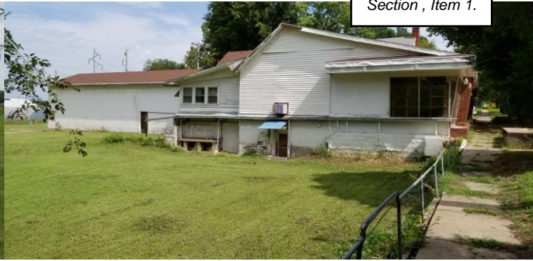
North side of property
