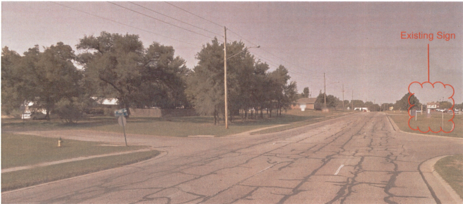
RADIO LANE LOOKING WEST
