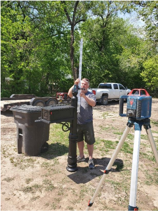
Bottom of stick shows required elevation in relation to mailbox
