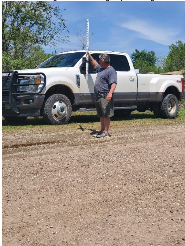
Bottom of stick shows required elevation at road level
