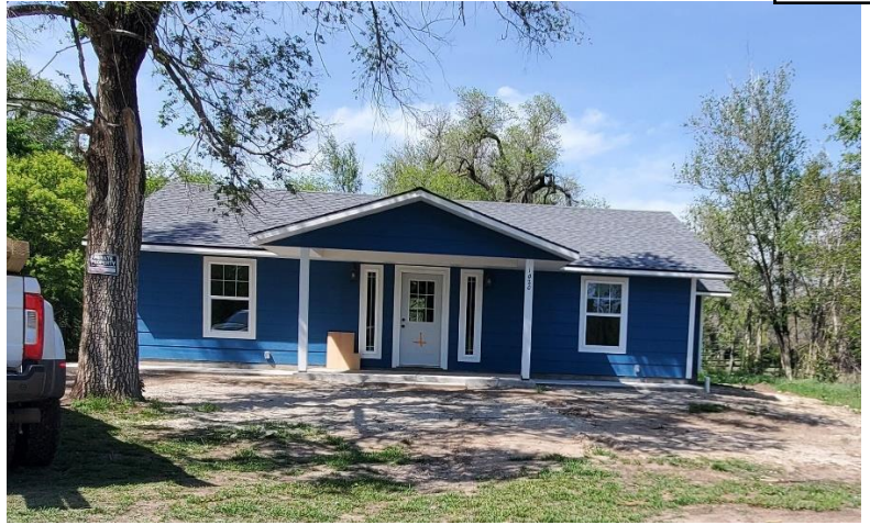
House with orange cross showing required height
