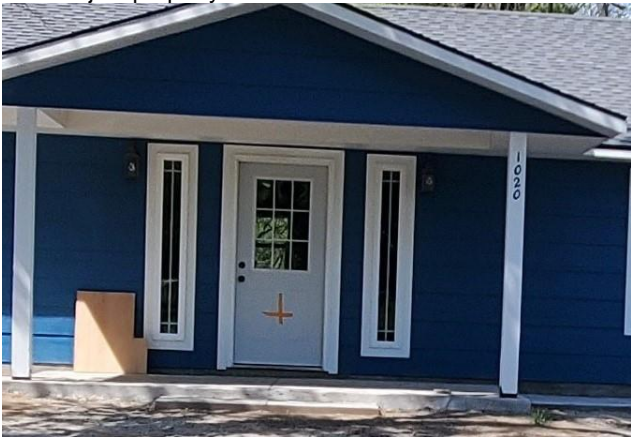
Close up view of orange cross marking required elevation
