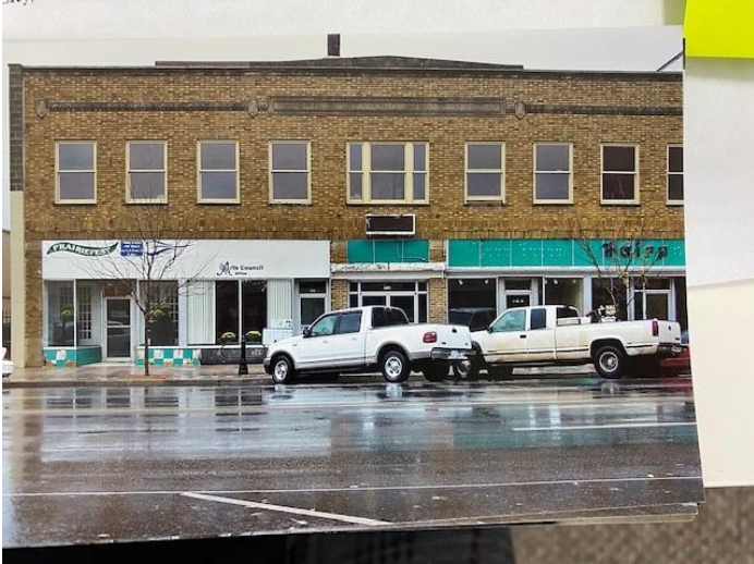
Undated photo provided by the Burford. It would have been taken shortly before the renovations began. The "sign board" existed at this time but it is likely that the windows were behind it as can be seen in the green panels to the south.
