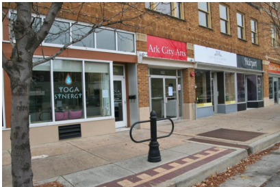
110-114 S. Summit. Storefronts looking south from north end. 11/14/2017. B. Spencer
