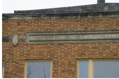
110-114 S. Summit. Detailing on parapet of west facade. 11/14/2017. B. Spencer
