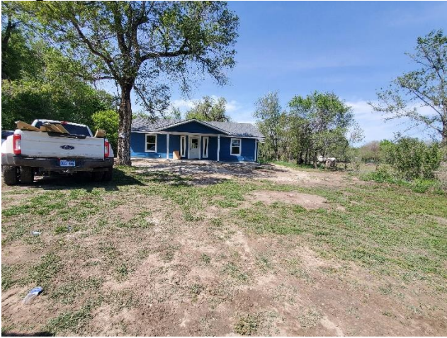
The subject property-1020 W 5 th Ave
