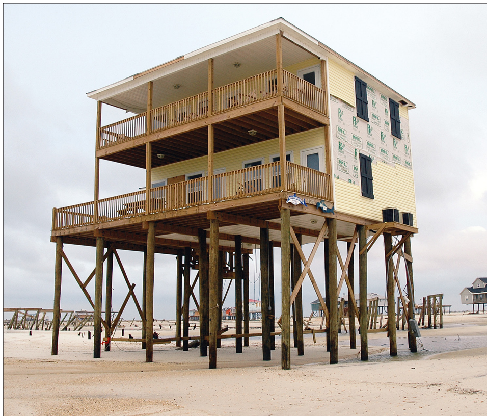
Figure 3-10. Home elevated on piles.
