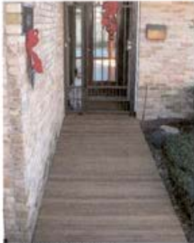
Over Old Concrete
