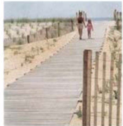
Sand Dune Preservation Modular Walkways.
