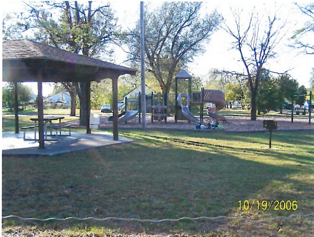
Park amenities such as the shelter, playground, BBQ grill are not on an accessible route.
