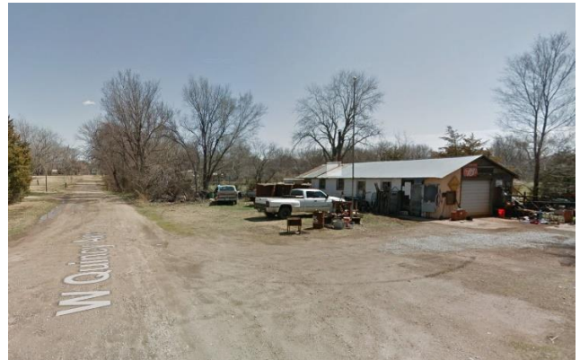
Welding Shop. Google StreetView from March 2014
