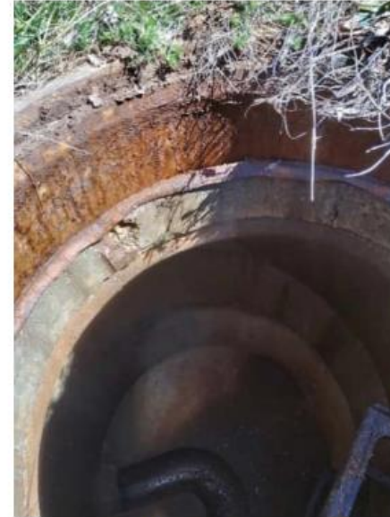
PS5-B-0018-MH: Install water-resistant manhole frame and cover & cementitiously line chimney
