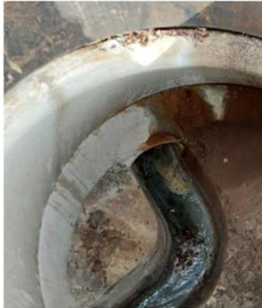
PS5-A-0001-MH: Seal precast joint
