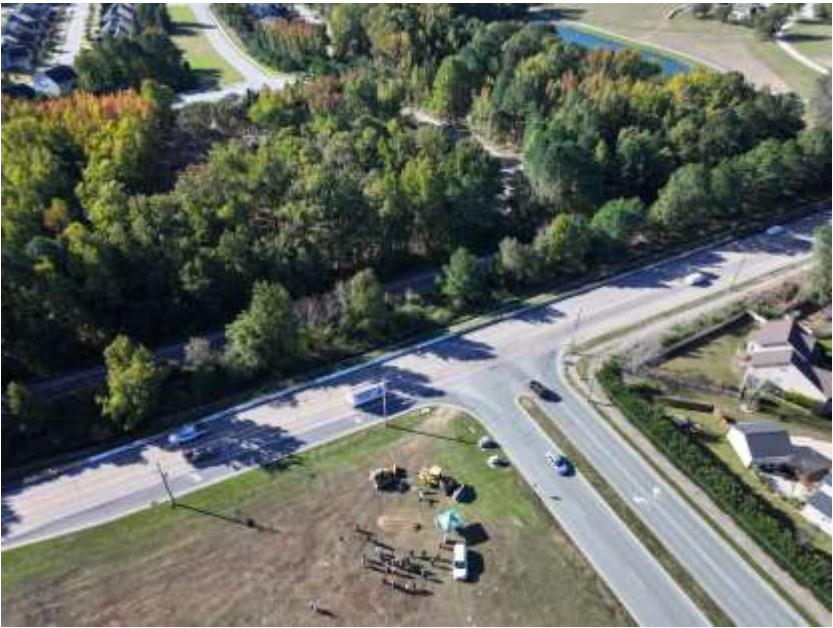
Apex Peakway Southwest Widening
