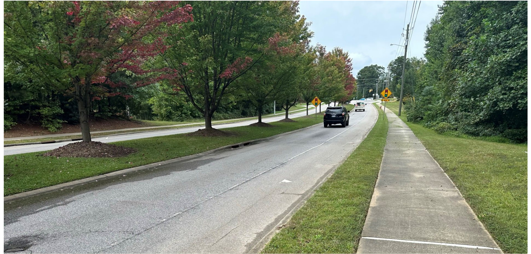
Existing typical section: 2-lane median divided with bike lanes and sidewalks
