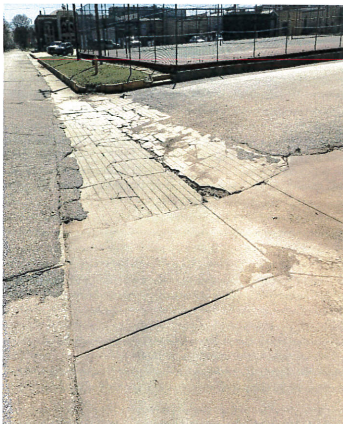
Corner of Anthony Ave. and Steadman St. looking south
