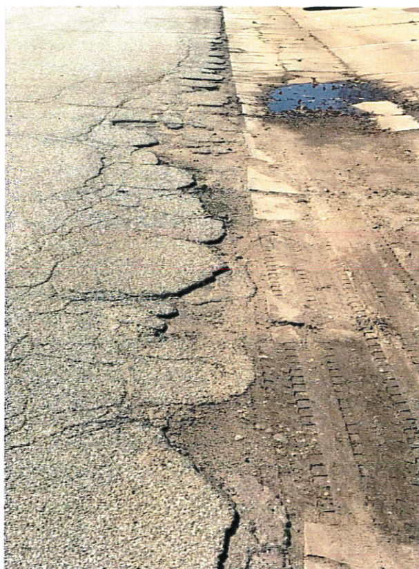
Corner of Steadman St. and Anthony Ave. looking west
