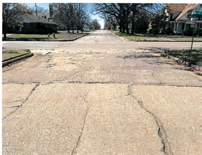
Corner of Spring St. and Jennings Ave. looking west
