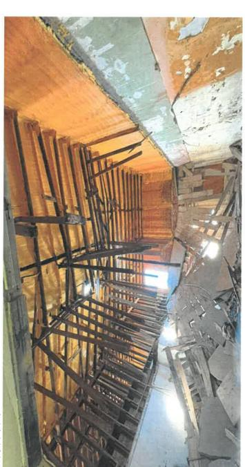
The Unsecure structures interior exists with a concrete floor approximately 4" thick has collapsed along with structural supports causing the roof to buckle and start collapsing. It does not appear to have any further supports for the brick walls other than the concrete holding the bricks together. The front of this structure faces Main St along a commonly used sidewalk.
