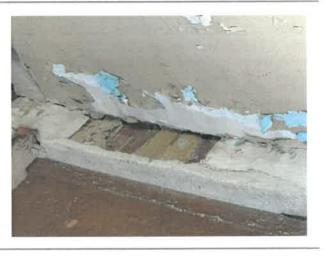
W Wall 206 daylight seen through cracks
