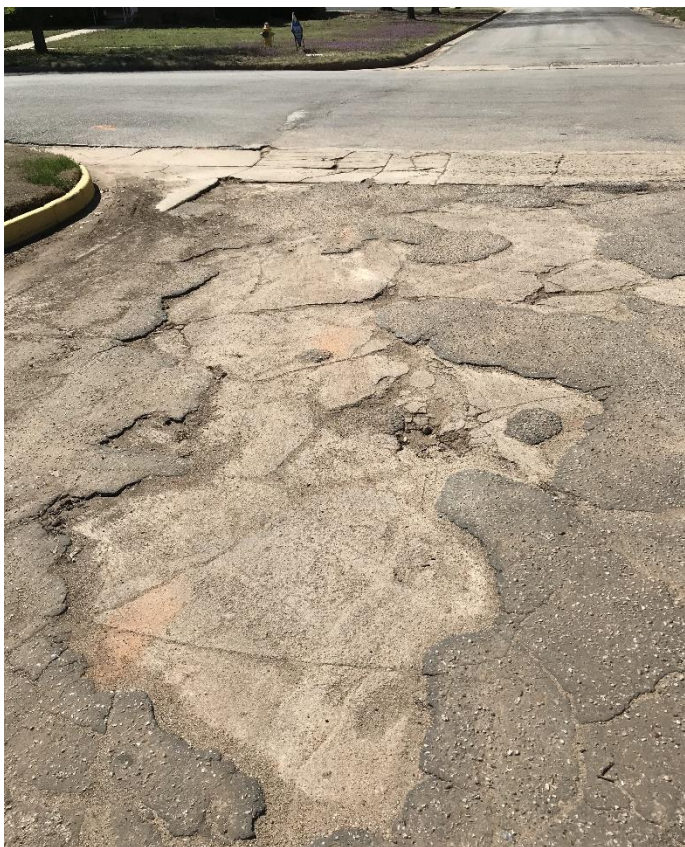
Corner of Spring St. and Jennings Ave. looking west
