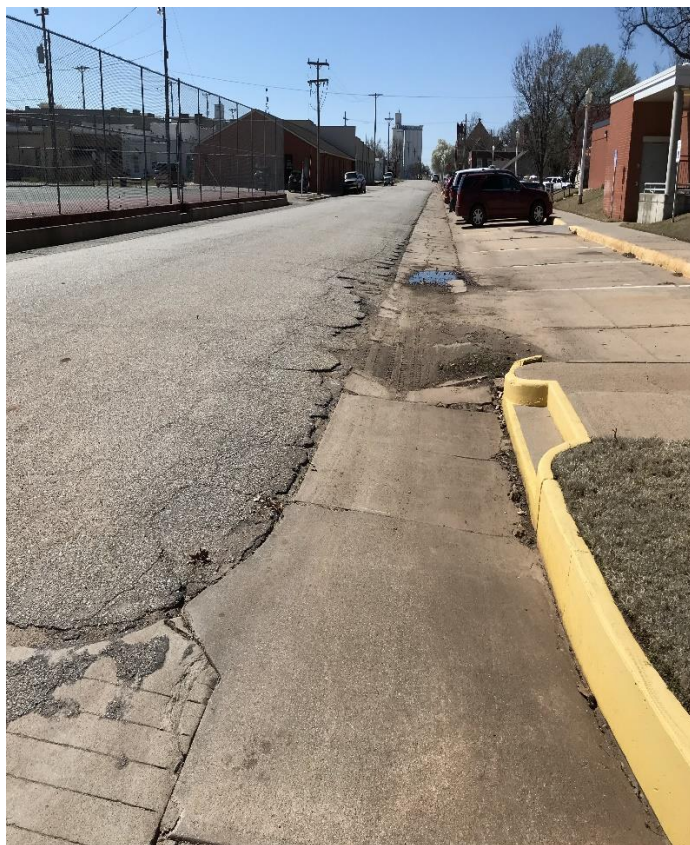
Corner of Steadman St. and Anthony Ave. looking west
