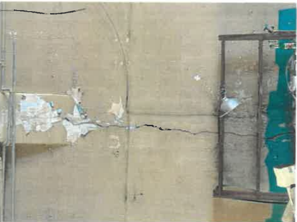
W Wall 206 daylight seen through cracks
