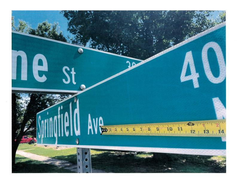
This is an example of TOO MUCH spacing between the end of the street name/Ave and the block numbers at the end of the sign. This sign did not need to be this long. Bid should only have spacing necessary to maintain overall minimum 30" sign length or a maximum length to fit the words with a maximum 4"gap between them.
