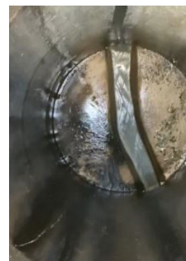
I&I from a joint in the MH
