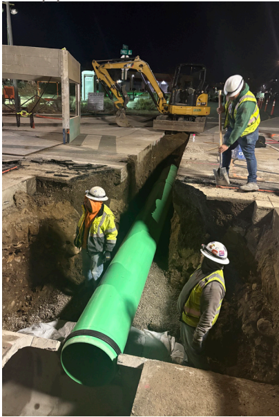
New pipe installation
