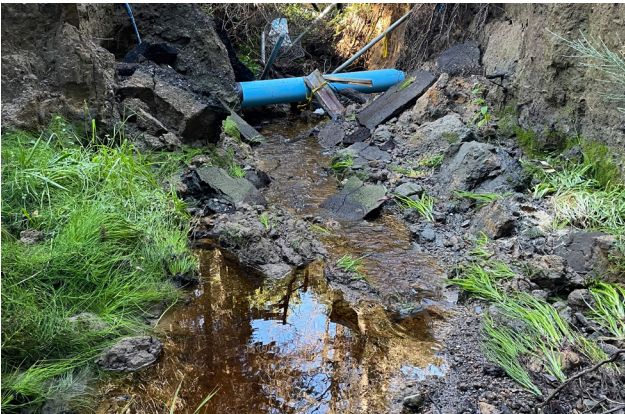
Brush Creek - Atmospheric River Culvert Failure
